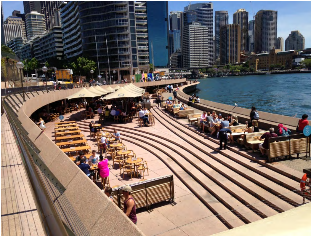
Photograph 1 – Existing Lower Concourse: View to the South
