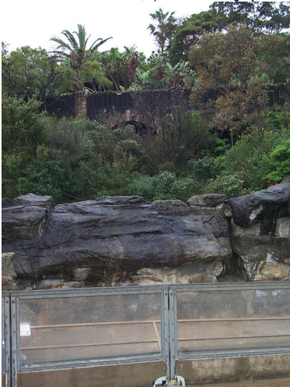
Figure 2.5.6.b View to a bridge crossing over the gully.
