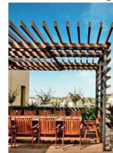
Steel framed hardwood timber shade structure
