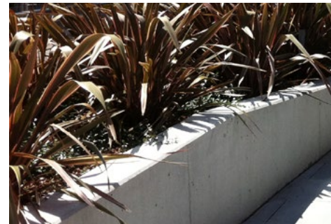
Potted plants and raised insitu concrete planters
