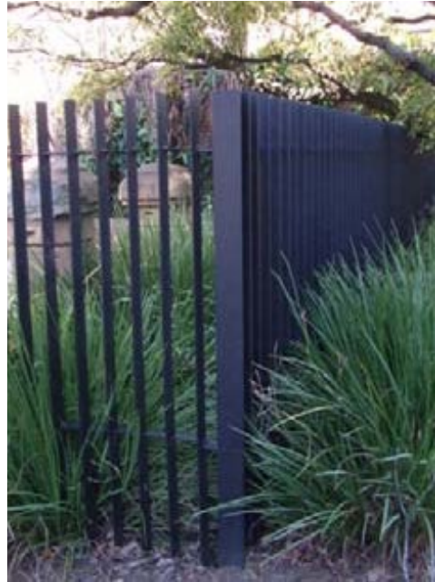
Steel palisade fencing
