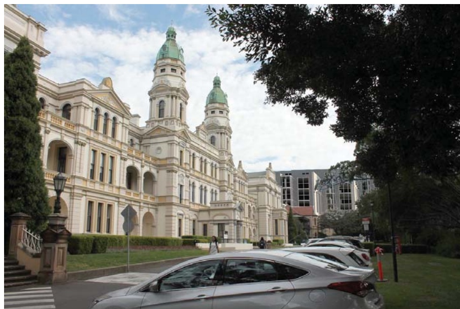
Internal Site View South towards Institute Building
