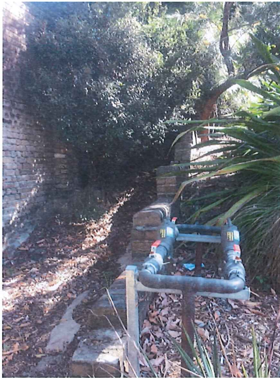
Photo - 13 Additionally wall construction and services on north face of wall
