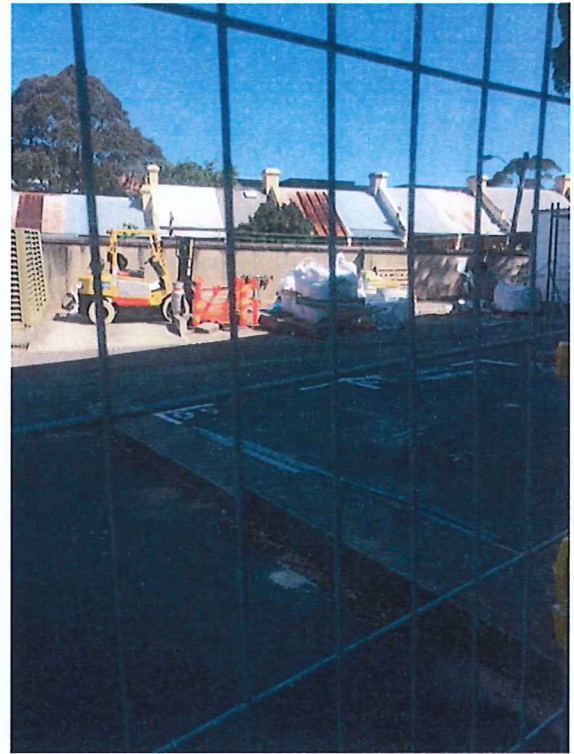
Photo - 14 Pavements on retained north face
