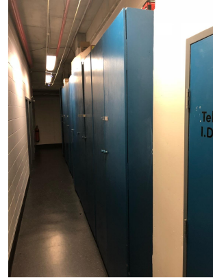
B003261-L8.2 Green top coat to blue undercoat Internal GF Walkway Timber built cupboards
