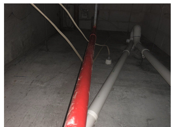
B003261-L3 Red top coat Internal B1 Whole Level Metal gas pipework throughout basement
