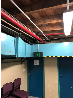
B003261-A2 Mastic Internal B1 Substage Mastic to metal ductwork
