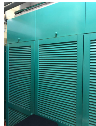
B003261-L8.3 Green top coat to blue undercoat Internal GF Laundry Room Timber built cupboards
