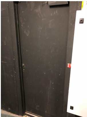
B003261-A3 Asbestos insulation board Internal B1 Orchestra Pit Door internal lining
