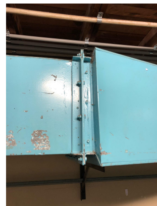
B003261-L5 Blue top coat to white undercoat Internal B1 Substage Metal Ductwork
