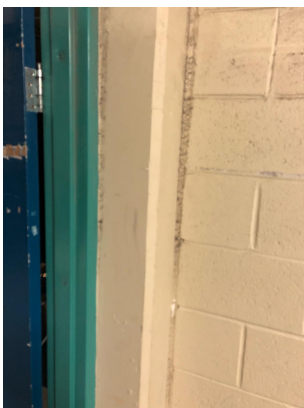
B003261-L1 Green top coat to brown undercoat Internal B1 Whole Level Door frames throughout basement
