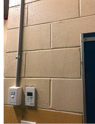
B003261-L9.2 Light yellow top coat Internal GF Laundry Room Walls high level
