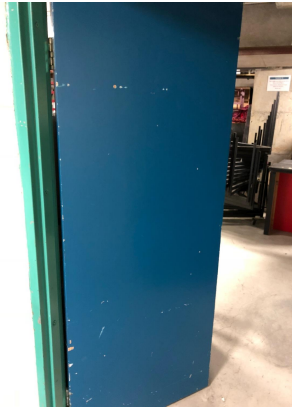
B003261-L2 Blue top coat to white undercoat Internal B1 Whole Level Doors throughout basement
