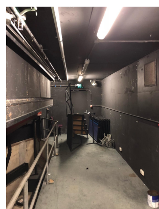
B003261-L6.1 Black top coat to red undercoat Internal B1 Orchestra Pit Walls & Ceiling
