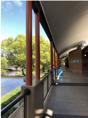
B003261-L24.2 Orange top coat External GF External Riverside walkway Metal structural beams
