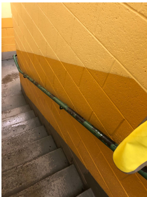
B003261-L8 Green top coat to blue undercoat Internal B1 Stairs to basement Metal Handrails
