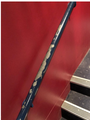
B003261-L20 Dark blue top coat to light blue undercoat Internal GF Fire exit lobby to courtyard Metal Handrails
