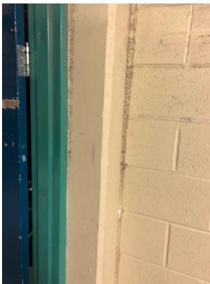
B003261-L16.1 Grey top coat with yellow undercoat Internal GF Lobby leading to courtyard Walls
