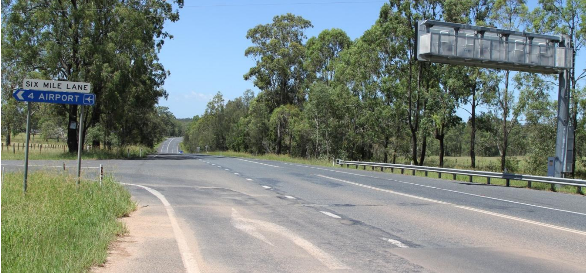
Figure 3-5 : Pacific Highway at Old Six Mile Lane (looking south)
