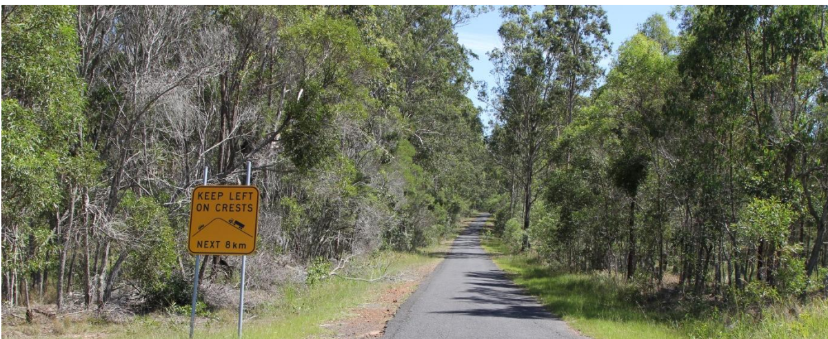
Figure 3-2 : Avenue Road (looking north of the Eight Mile Lane intersection)
