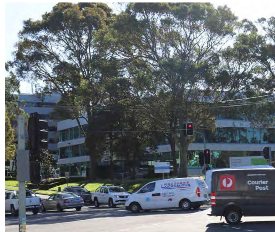
Figure 12 Existing commercial development on site.
