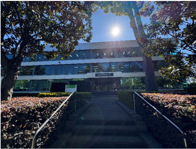
Picture 3 Existing commercial building at 4 Talavera Road, Macquarie Park from Talavera Road
