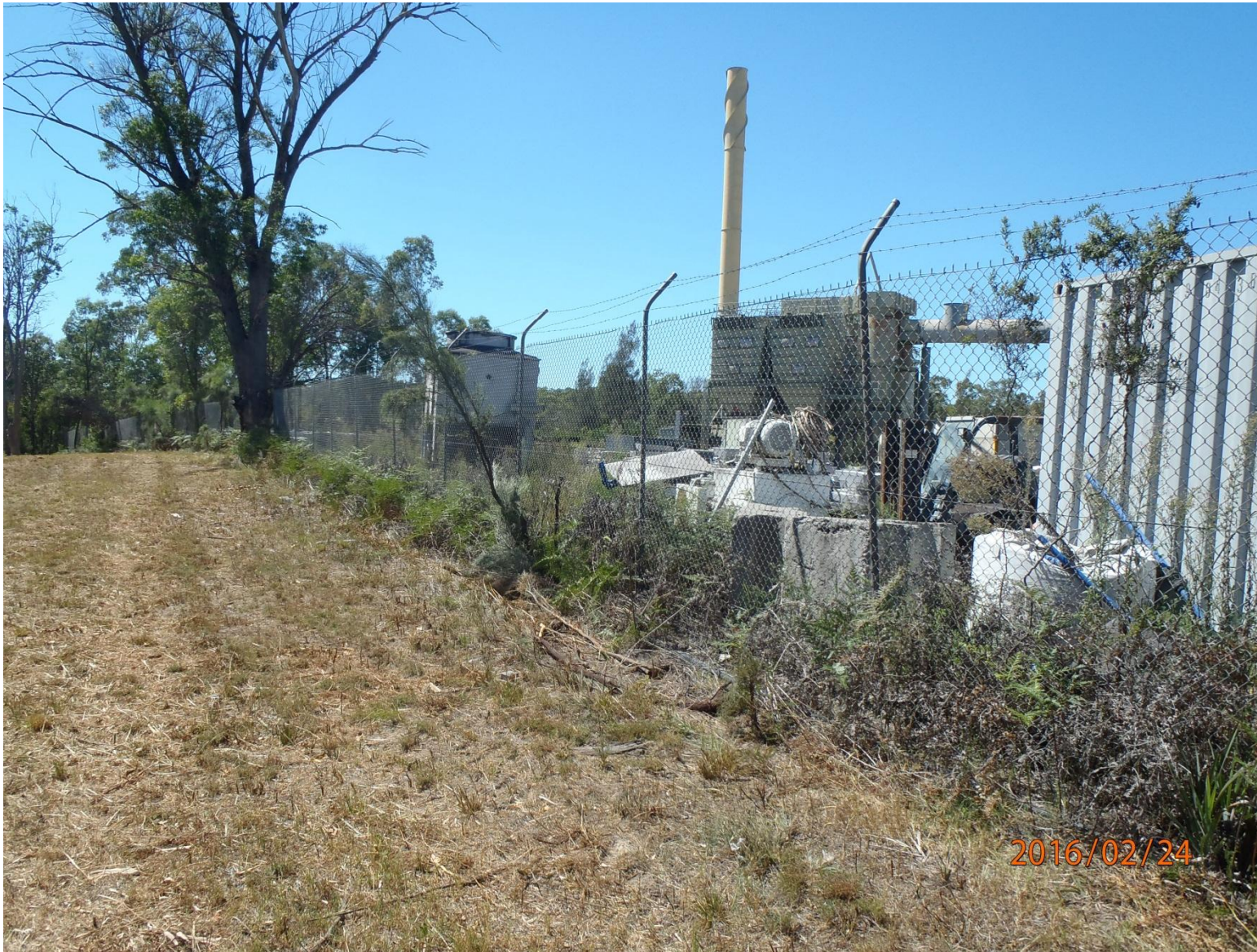
Plate 11 Northern Fence line and stored equipment within the proposed development footprint. Note: Baghouse 5 visible in the background.
