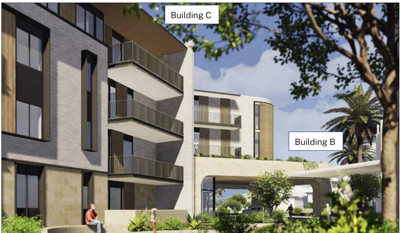
Figure 6 | Photomontages: view from Princes Highway to Building D (left) and Building E (right) with the heritage building at centre (TOP), internal view facing west to the port cochere and Building C (left) with Building B in the background (BOTTOM) (source: Applicant's documentation)
