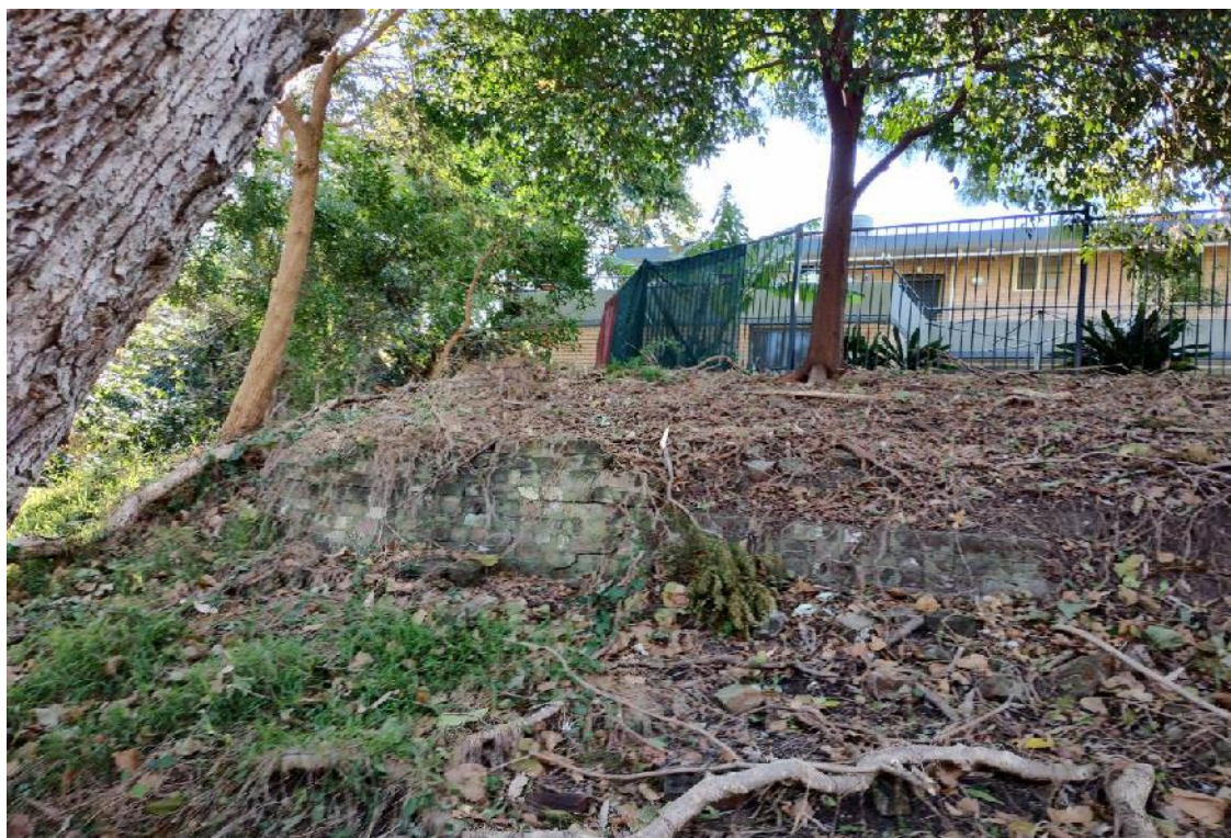
Photo 18: General view of south face of Blueberry Ash Village and former brick battering, looking north.
