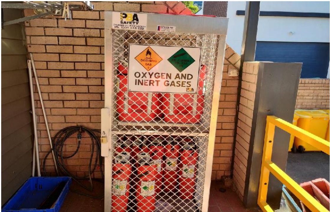
Photo 6: View of padlocked storage locker containing compressed oxygen in front of laundry in north western corner of the site, looking west.
