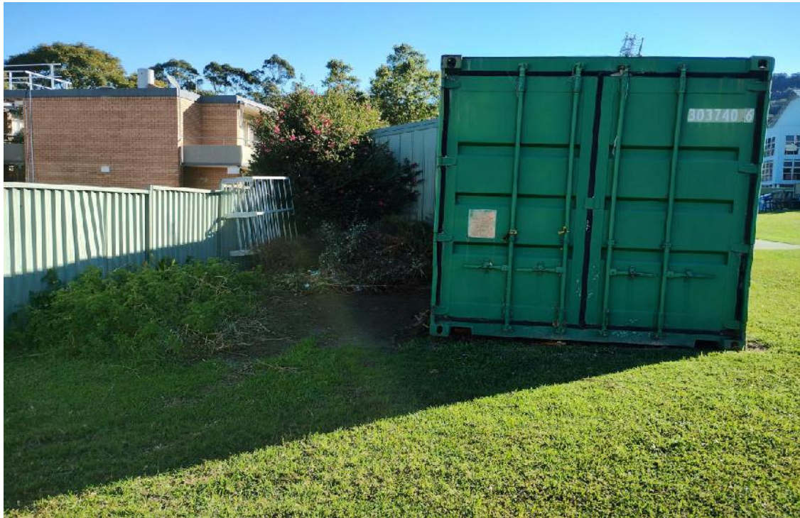
Photo 14: Storage container and tree debris storage area located east of main carpark, looking west.
