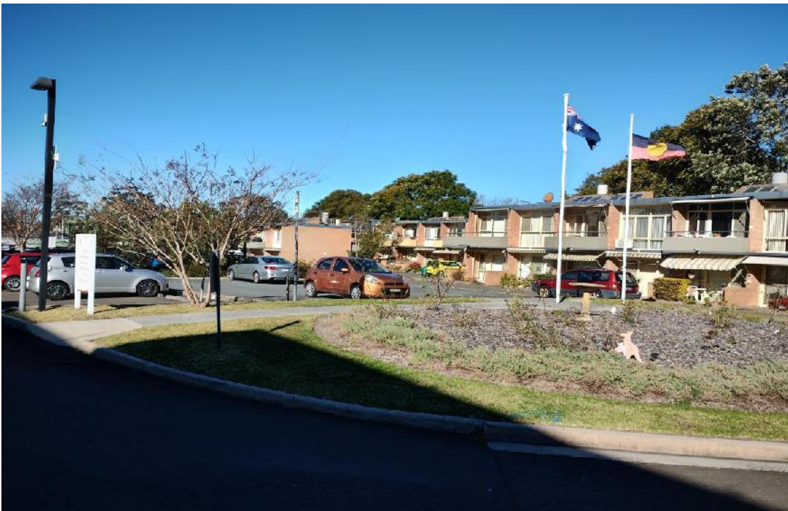
Photo 8: View of main hardstand carpark and residential building (Blueberry Ash Village), looking west.
