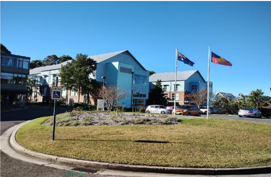
Photo 7: General view of gardens and residential building (Flame Tree Lodge), looking north east.
