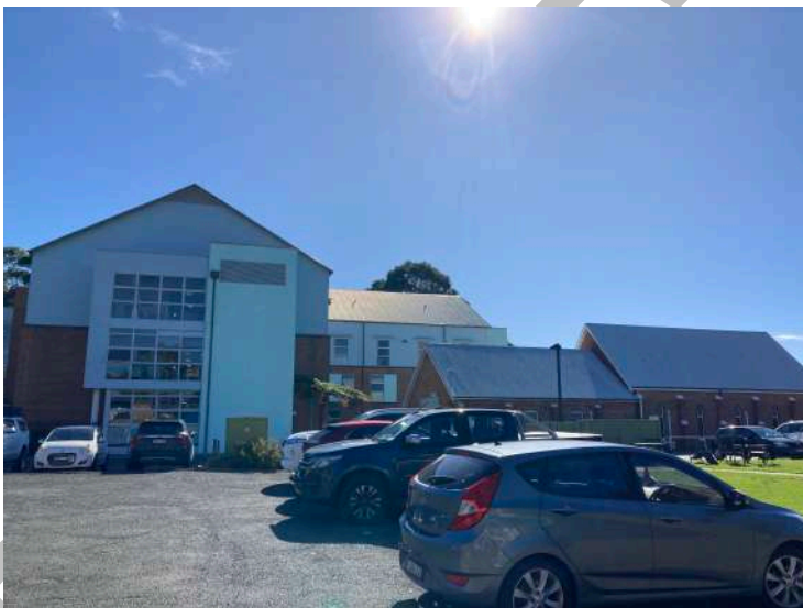
Figure 11: Photo of existing former Church south elevations.
