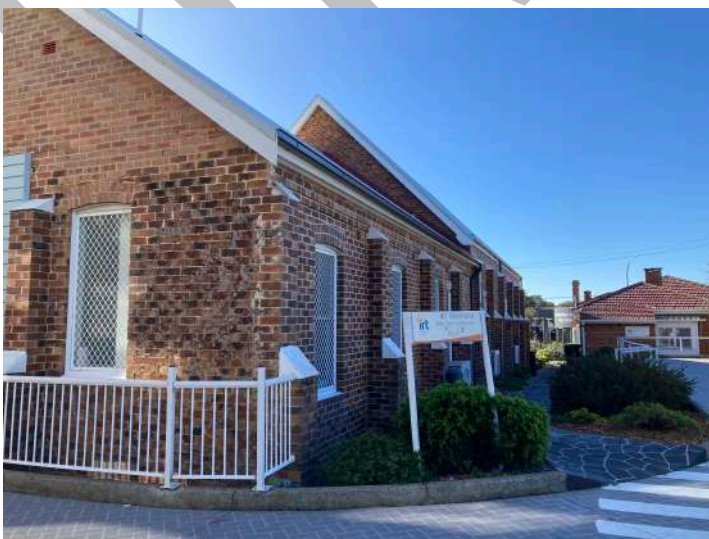
Figure 9: Photo of existing former Church west and south elevations.
