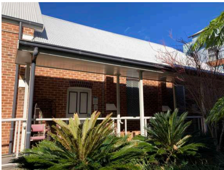
Figure 13: Photo of existing former Church north elevation. WPH.
