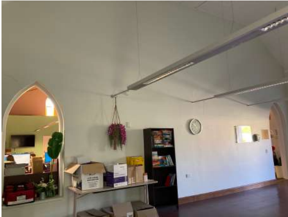
Figure 20: Photo of existing former Church Secondary Hall, looking west to rear.
