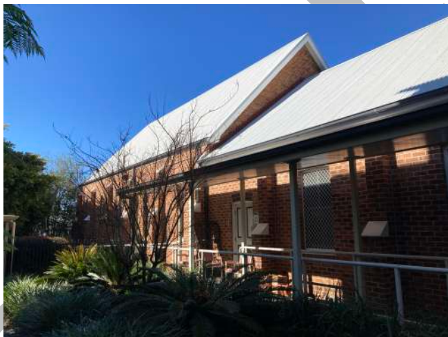
Figure 14: Photo of existing former Church north elevation. WPH.
