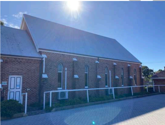
Figure 6: Photo of existing former Church south looking northeast WPH.
