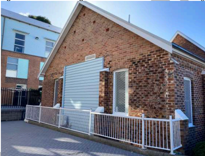
Figure 8: Photo of existing former Church west elevation looking northeast
