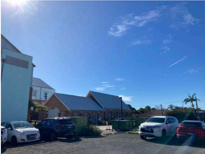
Figure 10: Photo of existing former Church west and south elevations.
