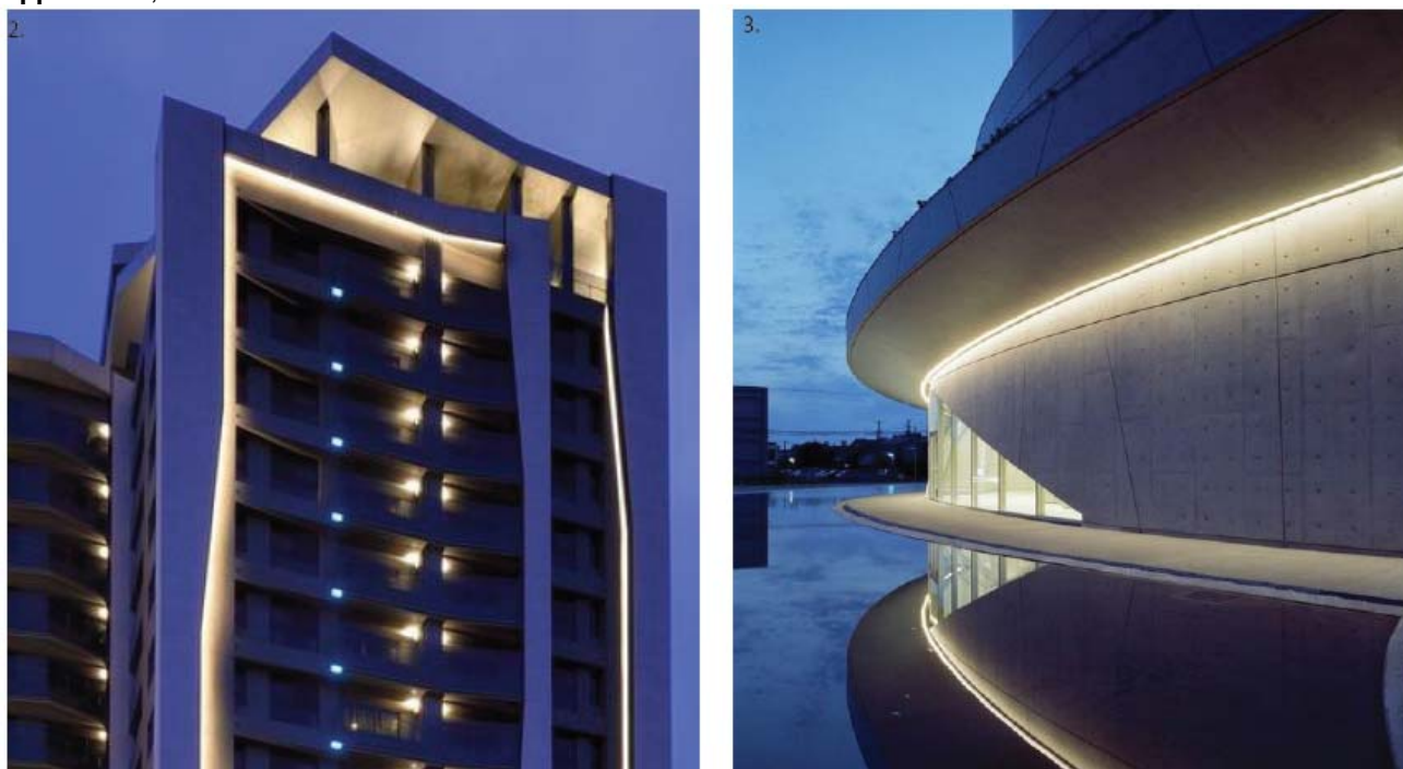
Figure 6 – Examples of façade lighting similar to that proposed under this Modification Application
