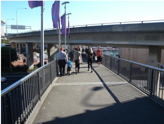
Figure 2.10: Pedestrian Overpass (looking west)
