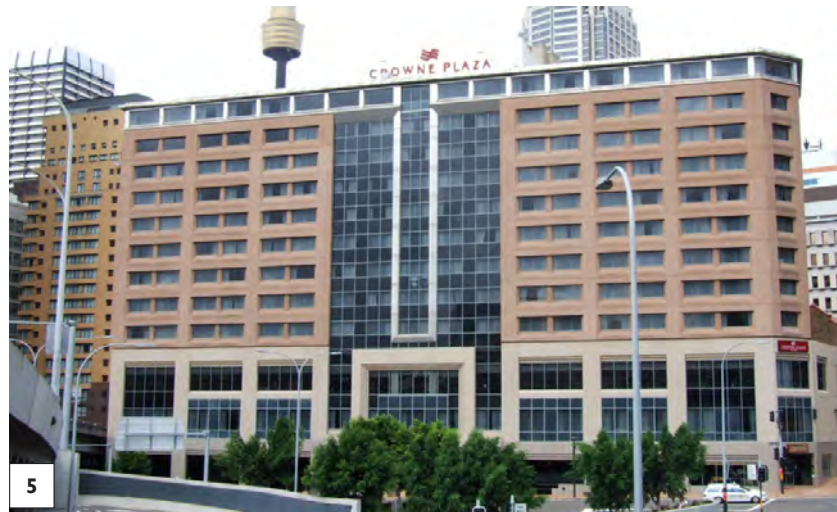
5 PARKROYAL Darling Harbour (eye level view from west)
