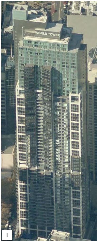
1 World Tower (bird's eye view from west)
