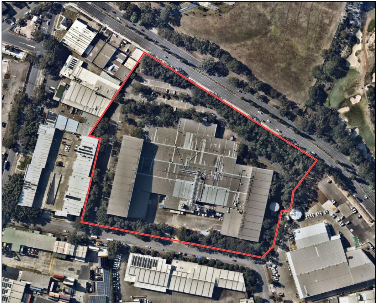
Figure 2: The Site (Source: Nearmap, 2024)
