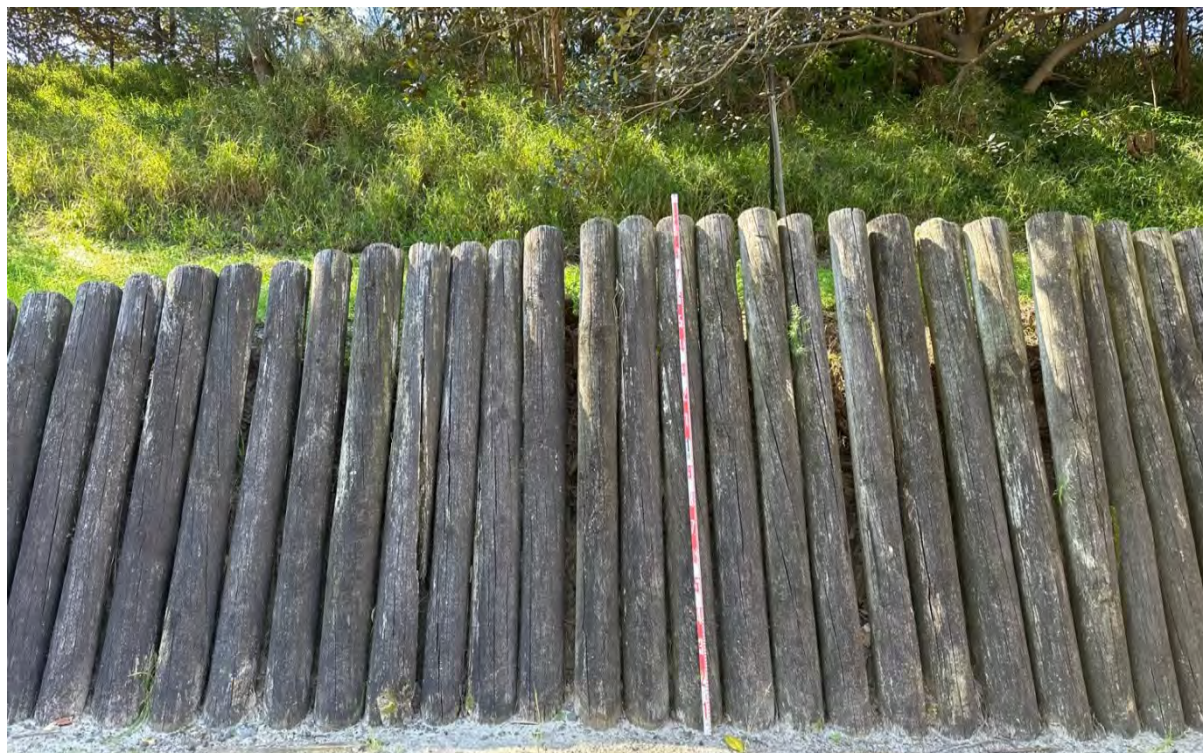
Figure 7.7 North facing view of current infrastructure within study area (2 m scale).
