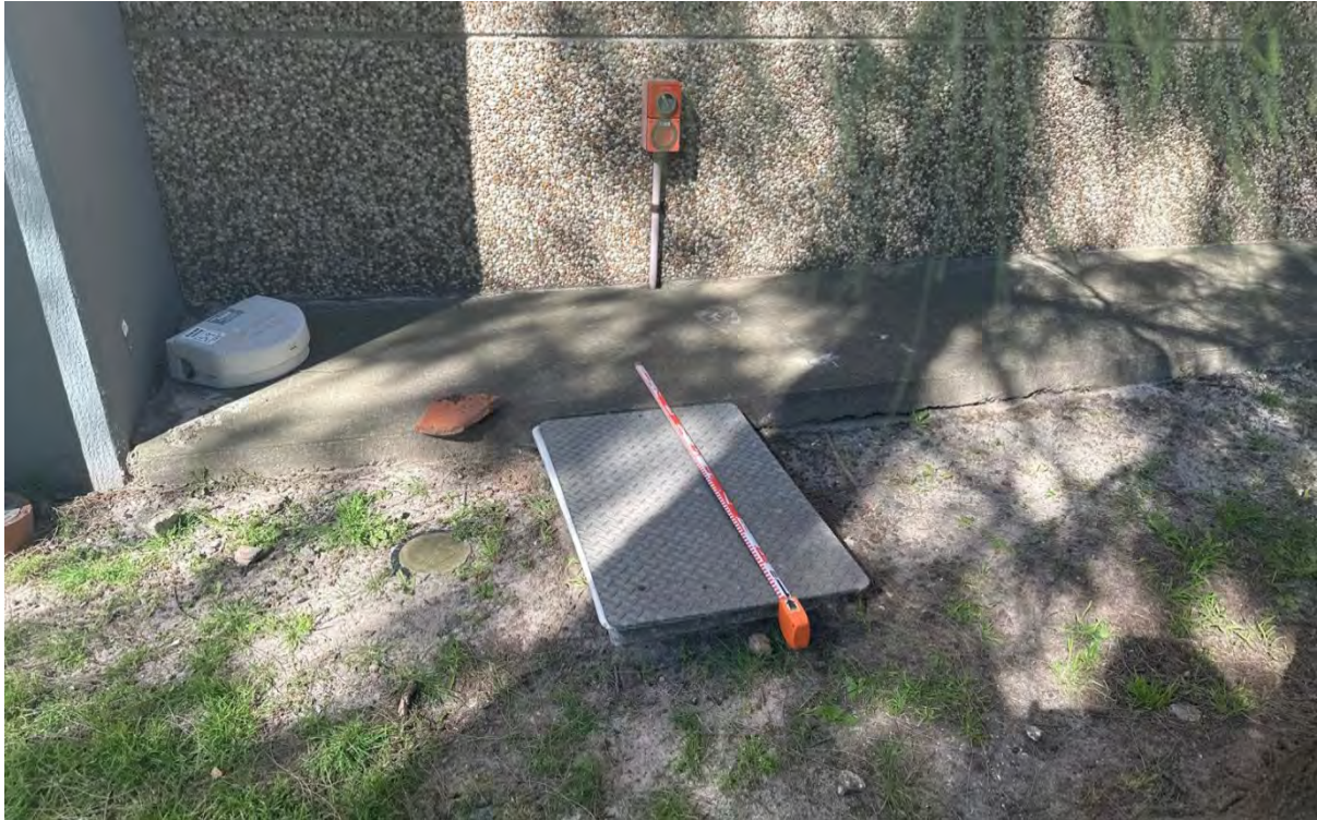
Figure 7.3 East-south-east facing view evidencing subsurface utilities and disturbance (1 m scale).
