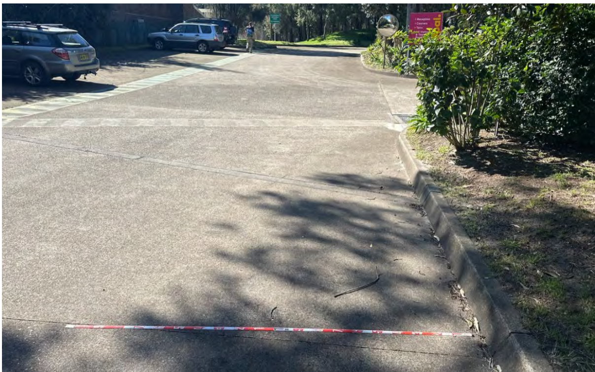
Figure 7.14 North facing view of concreted car park and access roads (2 m scale).
