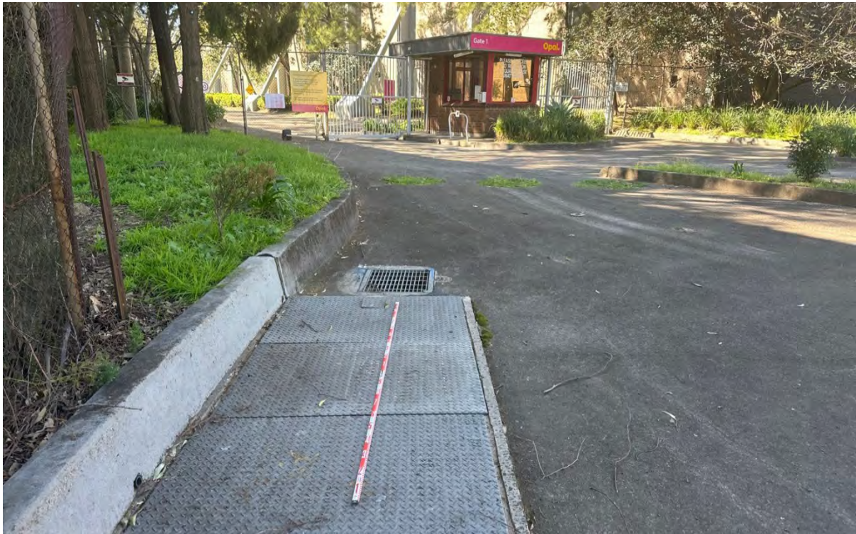
Figure 7.1 North-east facing view of concreted road and underground drainage (2 m scale).
