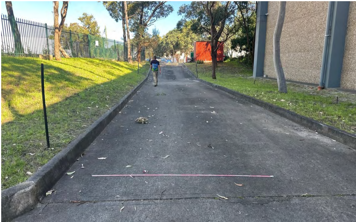
Figure 7.9 South facing view of concreted access road (2 m scale).
