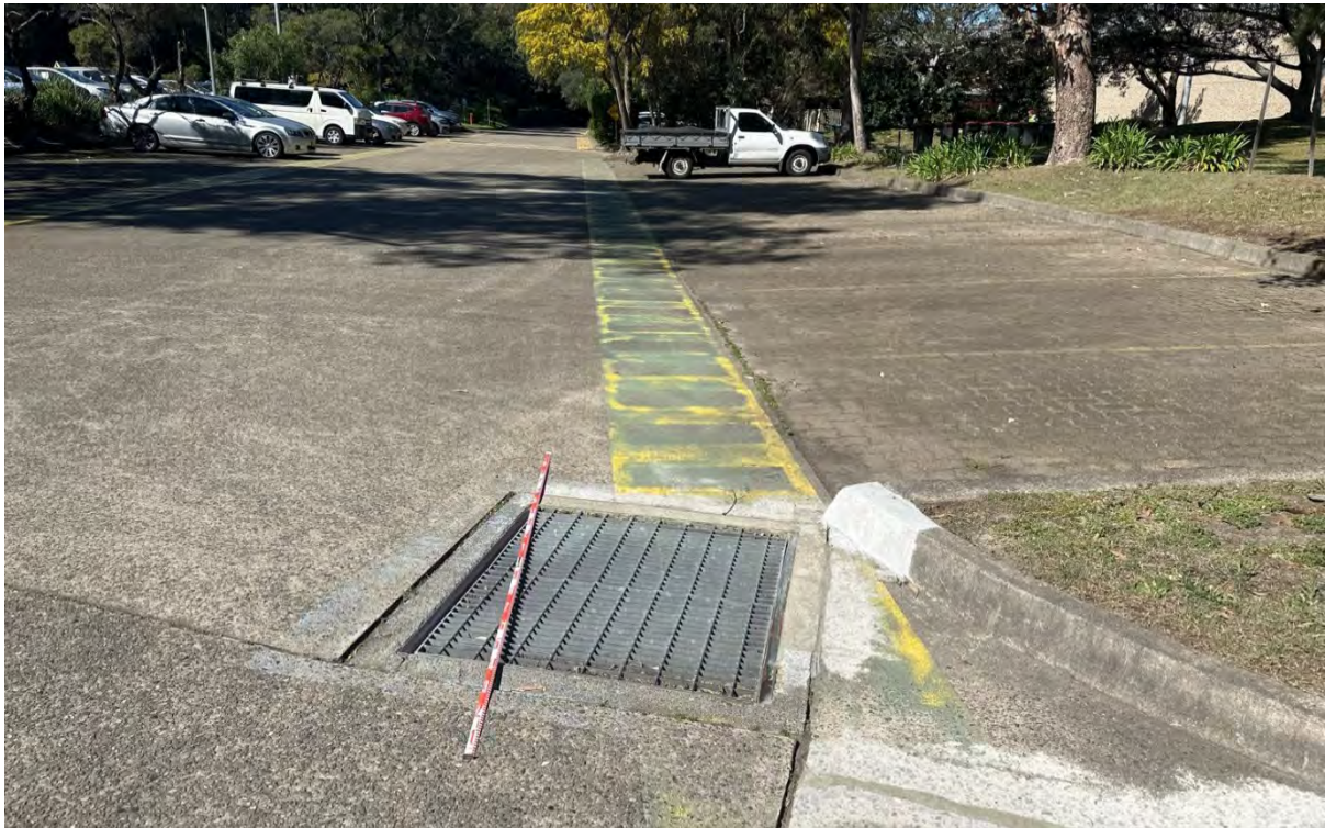
Figure 7.13 East facing view of underground drainage and paved car park (2 m scale).
