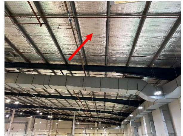
Photo 18: Main Warehouse – assumed SMF insulation to roof sarking
