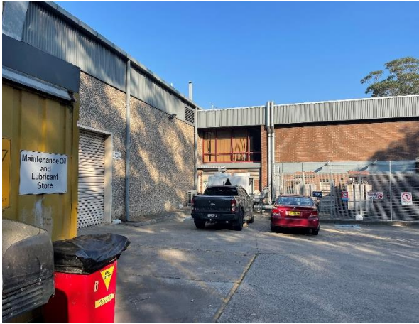
Photo 1: Overview of The Main Warehouse
