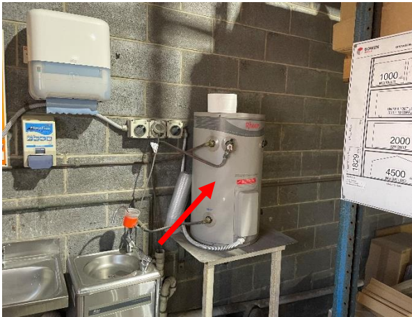
Photo 16: Main Warehouse – assumed internal SMF insulation to hot water systems
