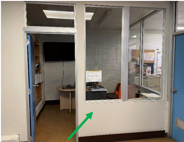
Photo 10: Main Warehouse – non-asbestos containing fibre cement sheeting to the mezzanine office walls in central portion
