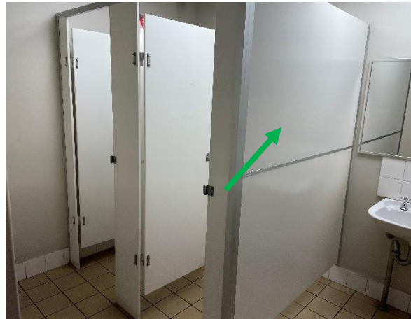
Photo 11: Main Warehouse – non-asbestos containing compressed fibre cement sheeting to the toilet cubicle walls and doors within the central portion
