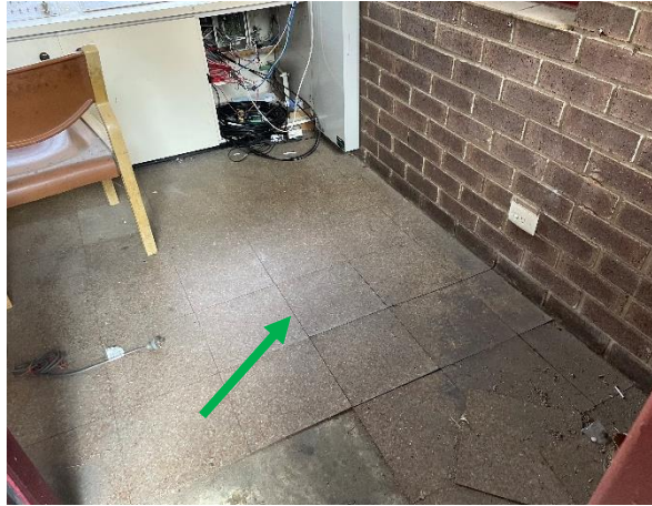
Photo 20: Gate House – non-asbestos containing red and green speckled vinyl floor tiles
