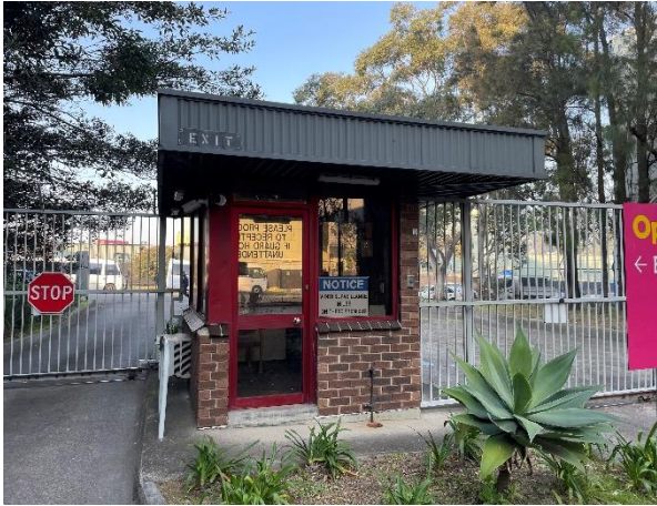
Photo 19: Overview of Gate House
