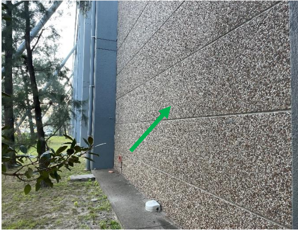
Photo 7: Main Warehouse – non-asbestos containing pebblecrete to the external walls
