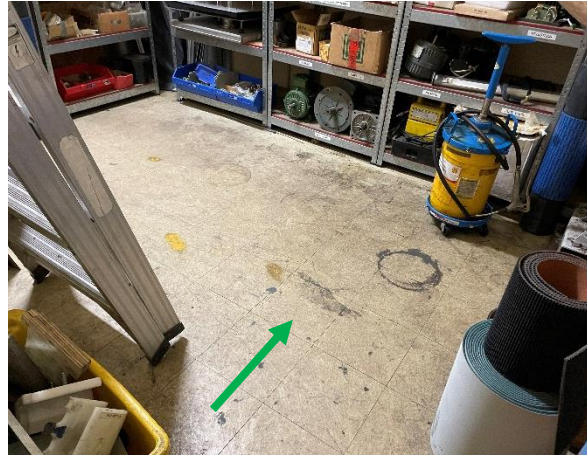
Photo 8: Main Warehouse – non-asbestos containing beige vinyl tiles to the floor of the store room within the central east portion
