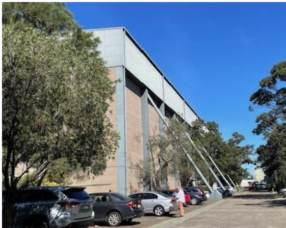
Current structure looking south to Moore St
