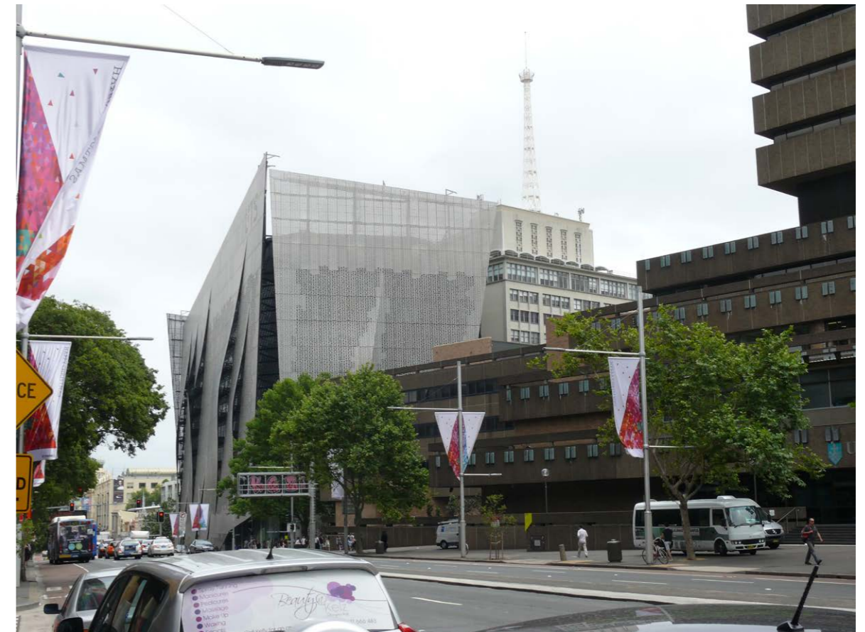
Photograph of existing view
