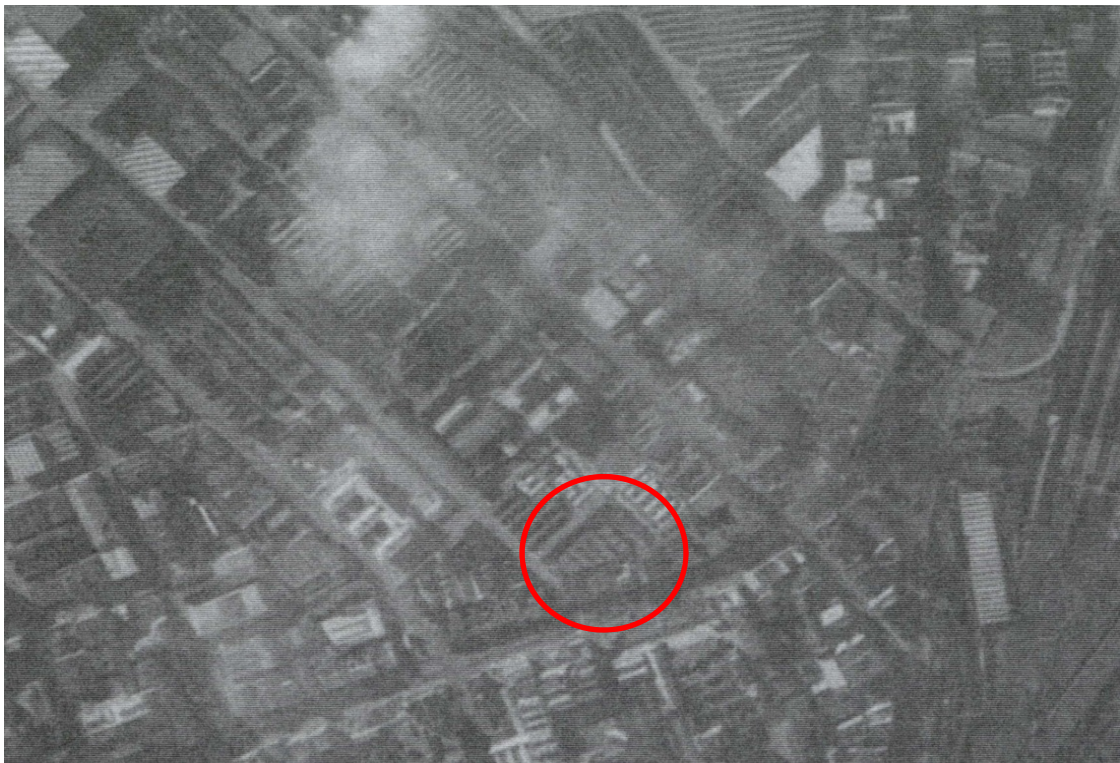
Aerial photograph from 1942
