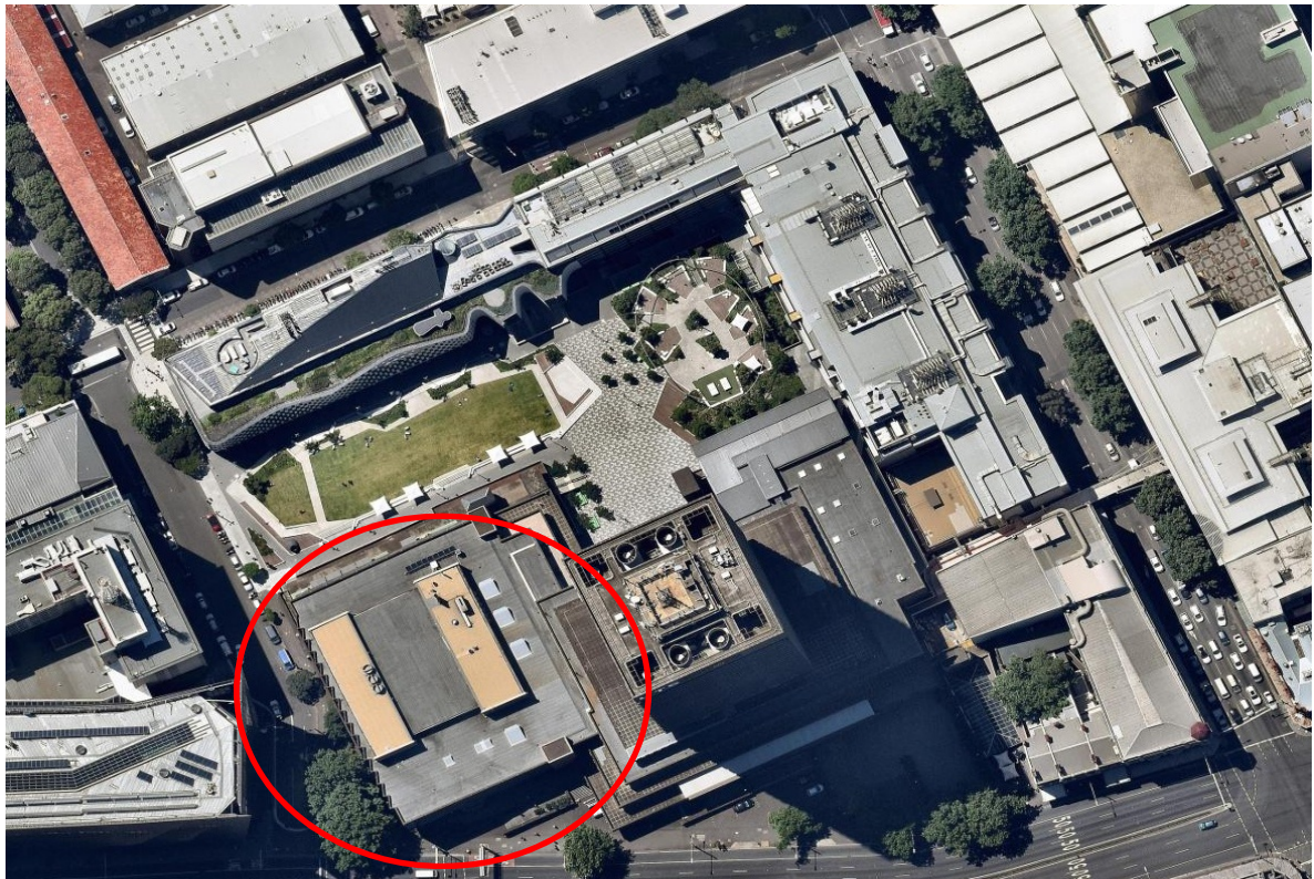
Aerial photograph from 2015
