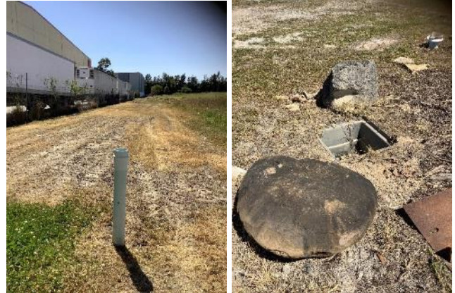
Figure 52. View to north and west respectively. Inspection of Survey Area 6, showing subsurface utilities, vehicle disturbance and dumped material.
