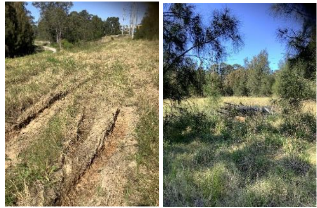
Figure 35. View to south and east respectively. Inspection of Survey Area 3, showing vehicle damage, dumped material and overgrown vegetation.
