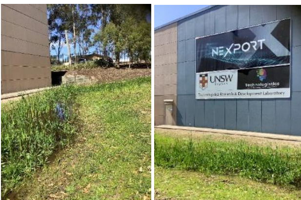
Figure 45. View to south and east respectively. Inspection of Survey Area 5 showing existing building and drainage channel and approximate location of 45-50483.
