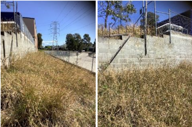
Figure 41. View to west and south respectively. Inspection of Survey Area 5, showing modified landscape.
