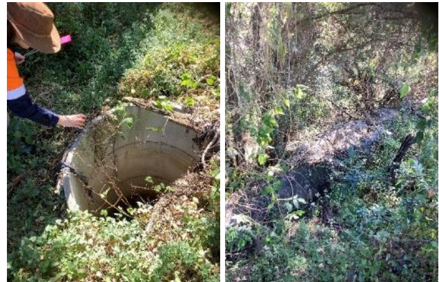
Figure 31. View to north. Inspection of Survey Area 2, showing subsurface drainage and overgrown vegetation surrounding sandstone retaining wall.
