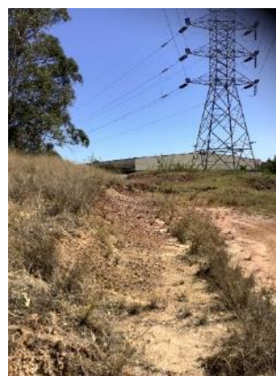
Figure 44. View to west. Inspection of Survey Area 5 showing vehicle damage, erosion and GSV.
