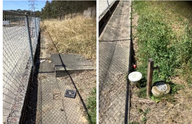
Figure 42. View to east. Inspection of Survey Area 5, showing subsurface utilities
