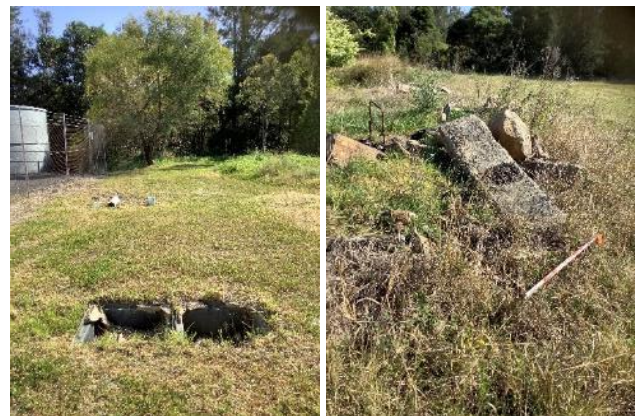
Figure 50. View to north and south respectively. Inspection of Survey Area 6 showing subsurface utilities and surface disturbances.
