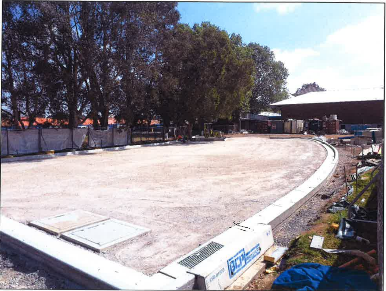
Figure 5: View looking at the O'Connell Street carpark (under construction).
