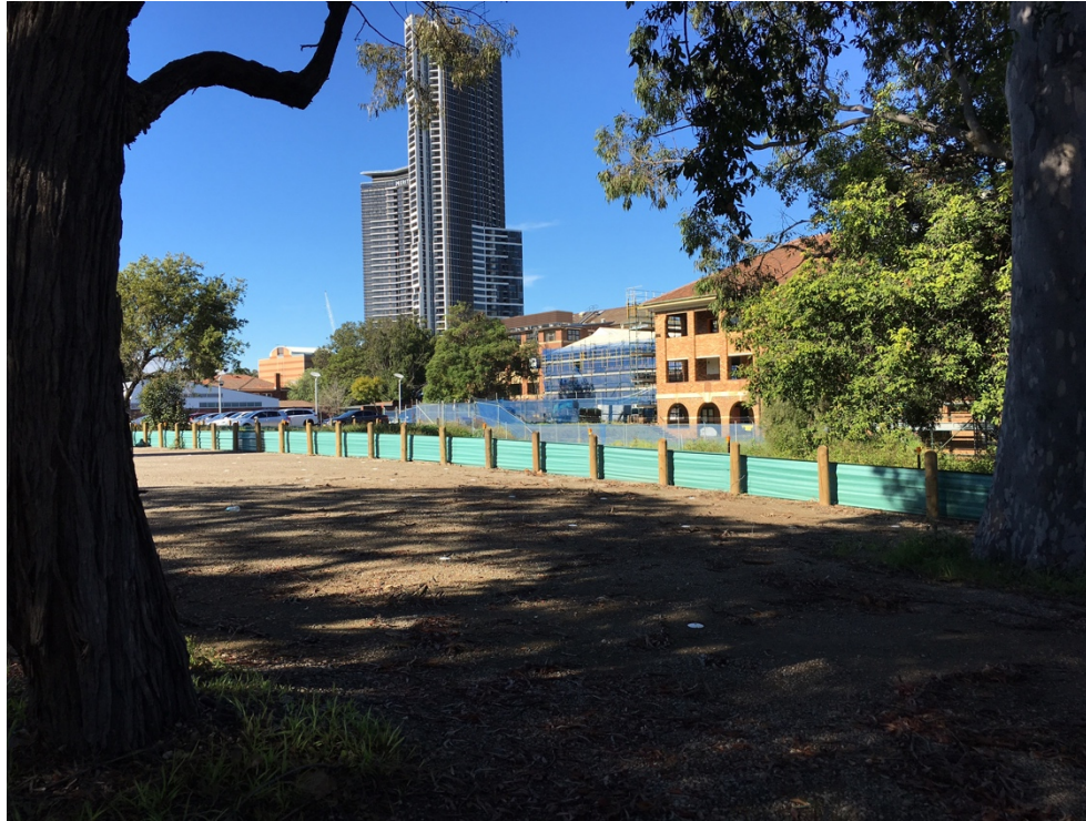
Figure11: View from Catholic Diocese Site, showing the minimal visual impact from the screened mechanical plant extension. A current DA Approval for the Catholic Diocese site will largely obscure views to the plant platform from the north and west. Source: TZG Architects, 2017.
