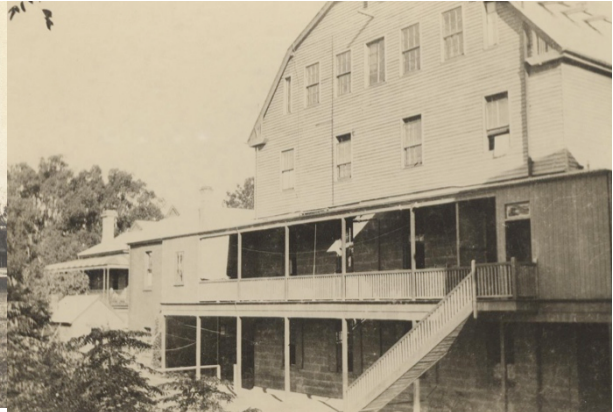
Figure 13: North side of Main School Block (Building B) showing additions, c1920. Source: King's School Archives.
