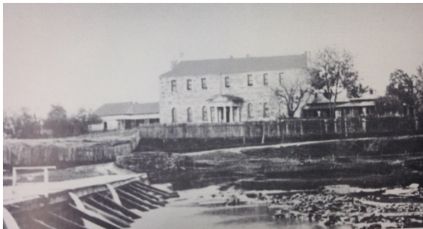
Figure 8: View of school from the river 1869, Lloyd Waddy, The King's School 1831-1981 , p73.
