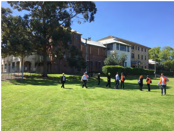
Figure 83: View to main building group from south west of Oval (prior to Early Works package demolition of structures in the courtyard of Group C, Building E, F and H).
