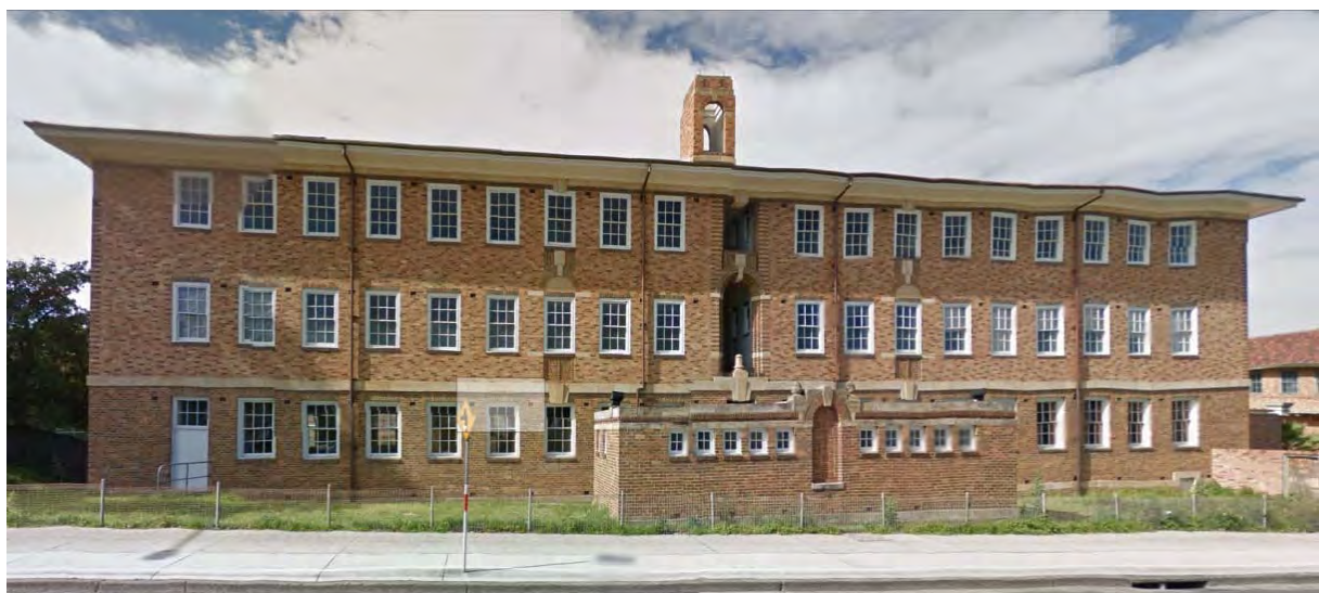
Figure 76: The O'Connell Street (western) elevation of Building D with single-storey toilet block at the front. (Source: Google street view).
