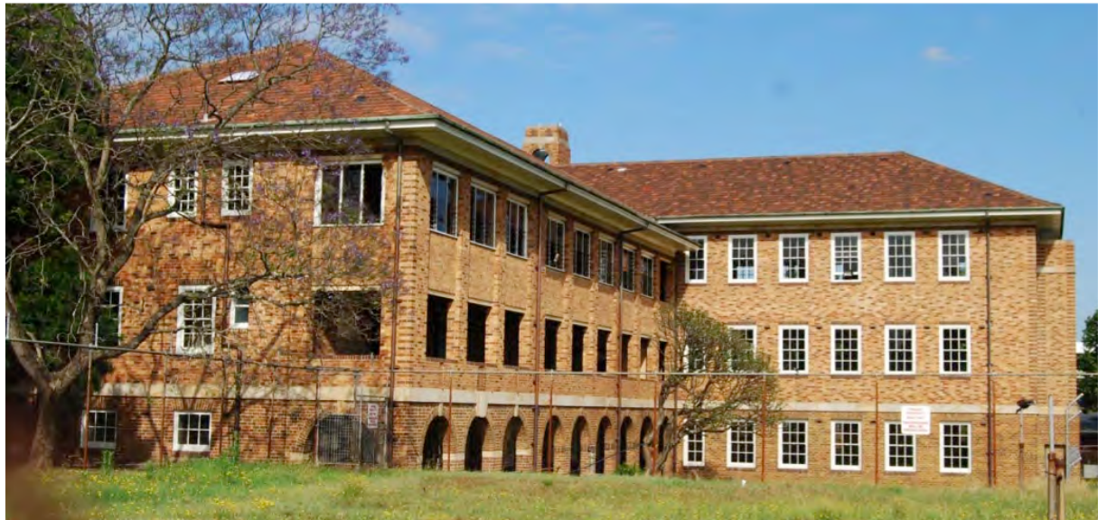
Figure 77: The rear north-east corner of Building D. The top floor of the balcony is enclosed. The different floor levels on the upper floors between the two wings of the building can be clearly seen. (Source: GAO)
