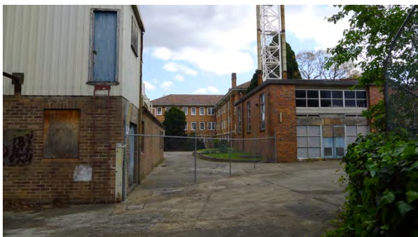
Figure 91: Concrete apron to rear of Building C and Building E (prior to Early Works package demolition of structures in the courtyard of Group C, Building E, F and H).
