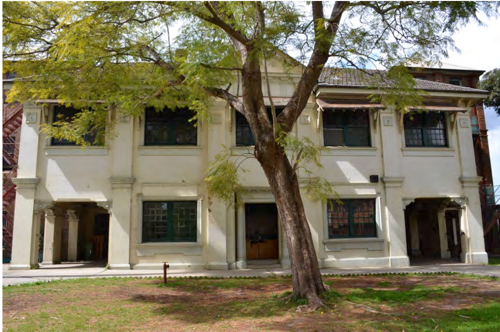
Figure 75: West face of Building C4. (Source: GAO)
