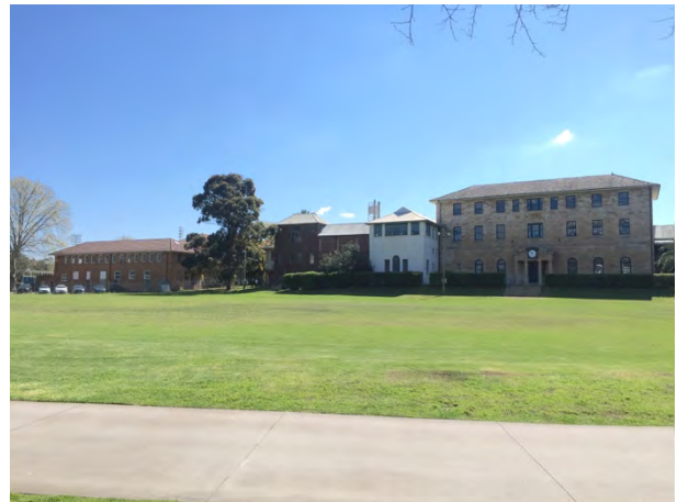
Figure 84: View to main building group from south of Oval (prior to Early Works package demolition of structures in the courtyard of Group C, Building E, F and H).
