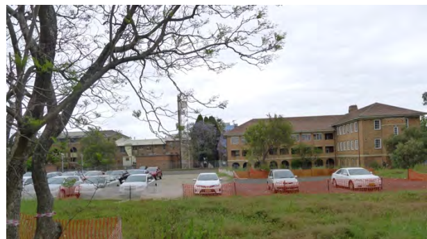
Figure 92: View to rear of Building D from neighbouring site (prior to Early Works package demolition of structures in the courtyard of Group C, Building E, F and H).
