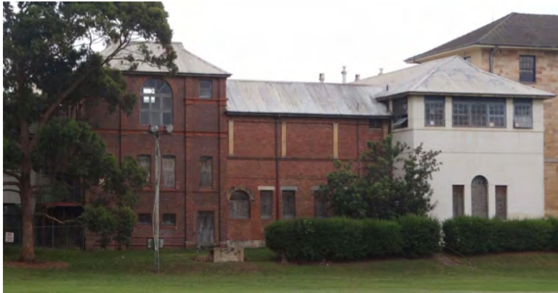
Figure 74: South face of Building C3. The two storey dining hall (white rendered building on right) was built first, followed by the three storey building on the left hand side. The central connecting building was the last completed. As a consequence, this wing is the most problematic for level differences across floors.
