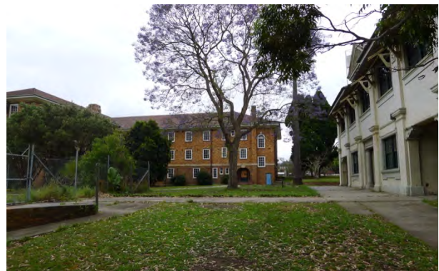
Figure 90: Courtyard between Buildings C, D and F.
