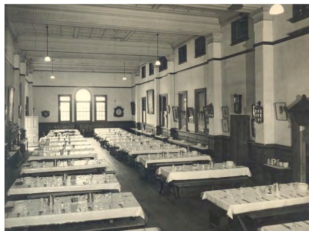
Figure 72: Former Dining Hall. Source: GAO, 2015
