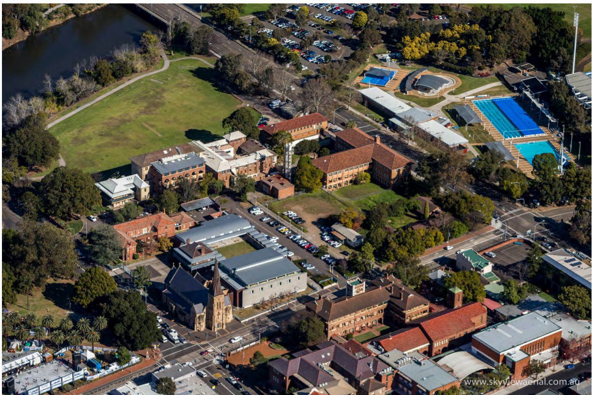
Figure 81: Aerial of the site viewed from the north (prior to Early Works package demolition of structures in the courtyard of Group C, Building E, F and H).
