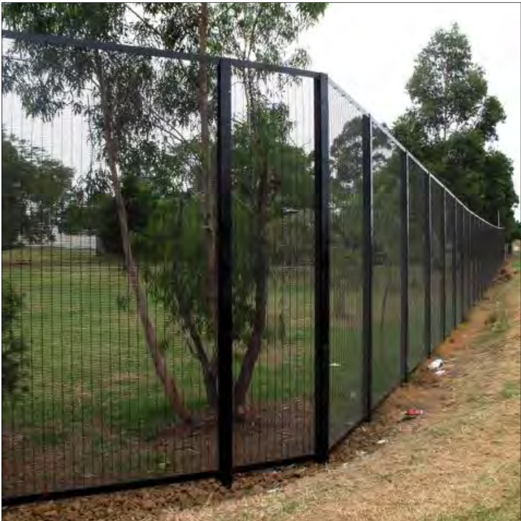
PMS MESH FENCE AT COLYTON PUBLIC SCHOOL
