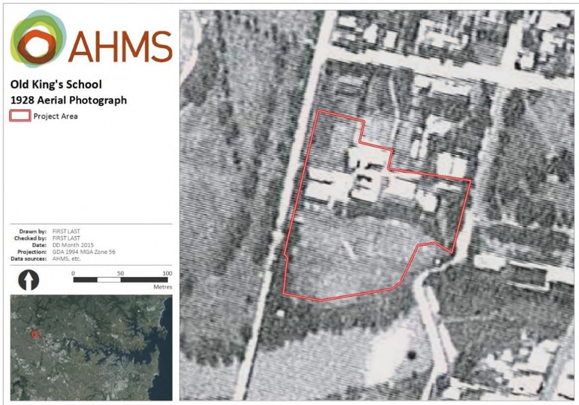
Figure A3-25. 1928 aerial photograph (Source: NSW Department of Lands).
