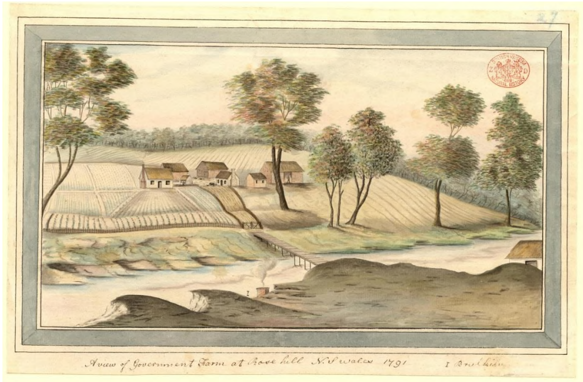
Figure A3-1. Government Farm, 1791 by a “Port Jackson Painter”. Subject area at extreme right
