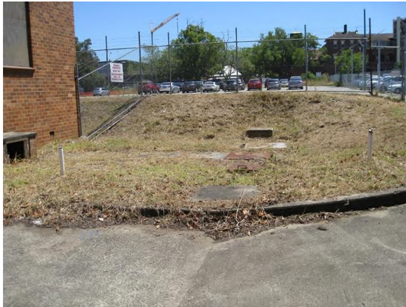
Figure 10 Cut on northern side of Building E (Boiler House), looking north.
