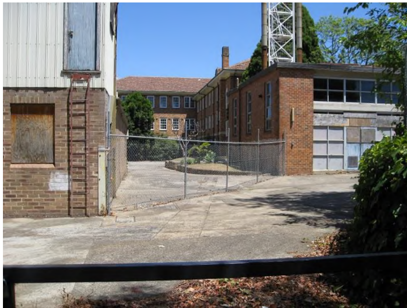
Figure 9 Northern portion of the site Building E (Boiler House) at right, Building C at left and Building D in distance (looking west).
