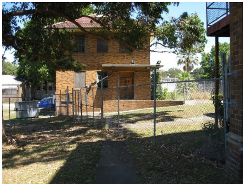
Figure 13 View west from front of main building. Building C at right, Building F in centre, Building G at far left.
