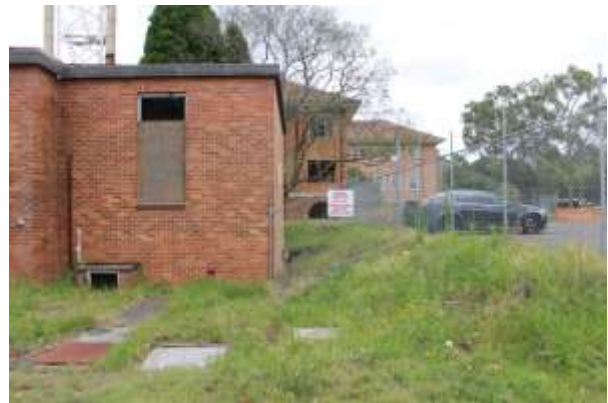
Plate 4. View west showing extensive cutting back along northern boundary of subject area, Boiler House, northern portion.
