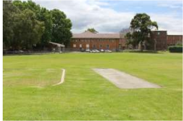
Plate 8. Concrete pad and irregularly shaped footing within playing fields, central portion.
