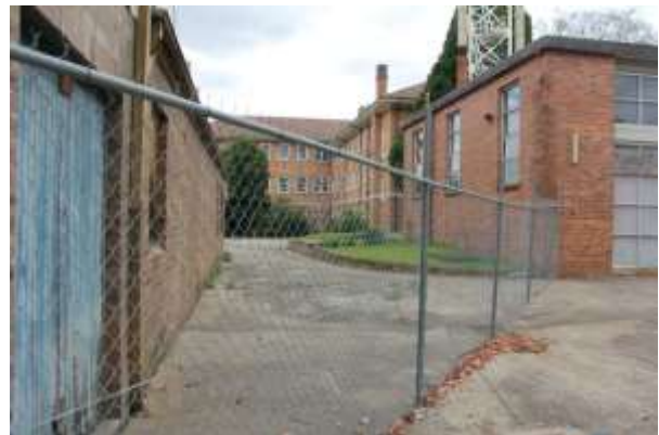
Plate 12. Concrete slab flooring and existing structures, northern portion. Note brick retaining wall as evidence for substantial levelling and filling.
