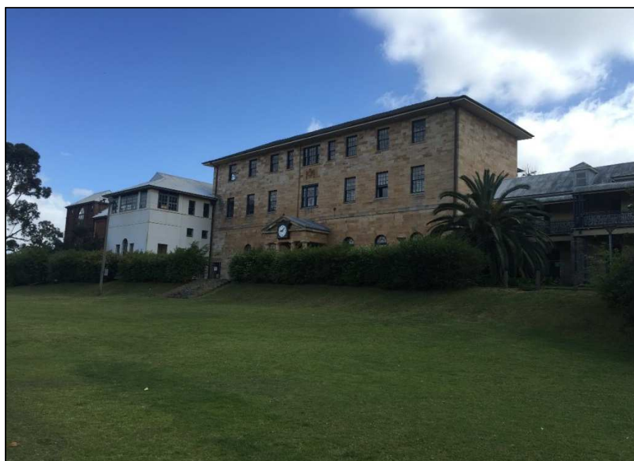
Figure 4: View north toward Building C (left), Building B (centre), Building A (right) and oval
