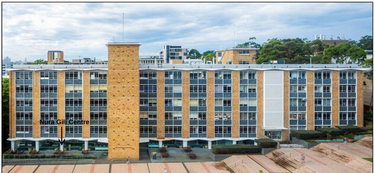
Figure 6 – Current view of South Block looking north
