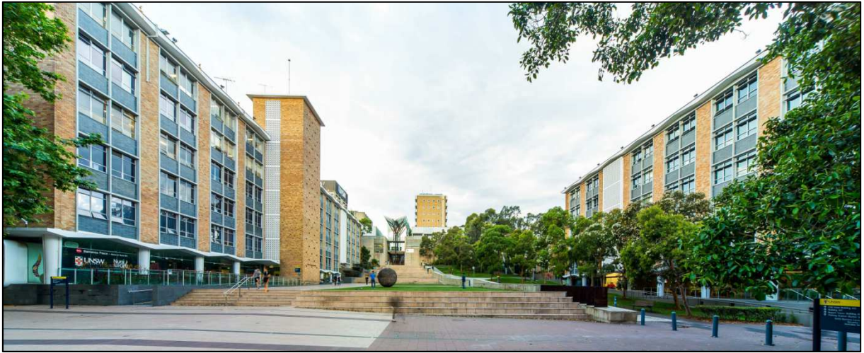
Figure 4 – Existing EEB building (on left) looking east towards the John Niland Scientia Building (source: Applicant's EIS)
