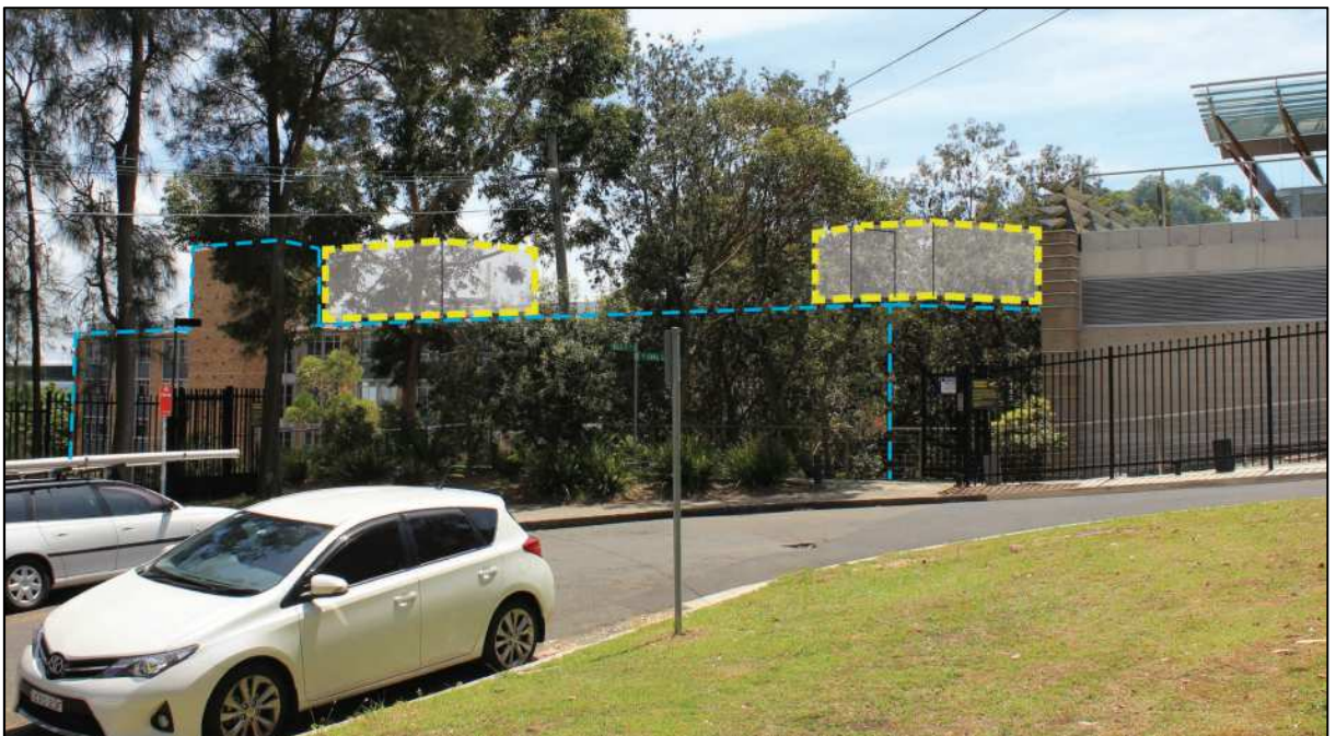
Figure 16 – View of EEB from corner of Willis Street and Oval Lane looking north-west, envelope of proposed additional rooftop plant shown in yellow. (source: Applicant's EIS)
