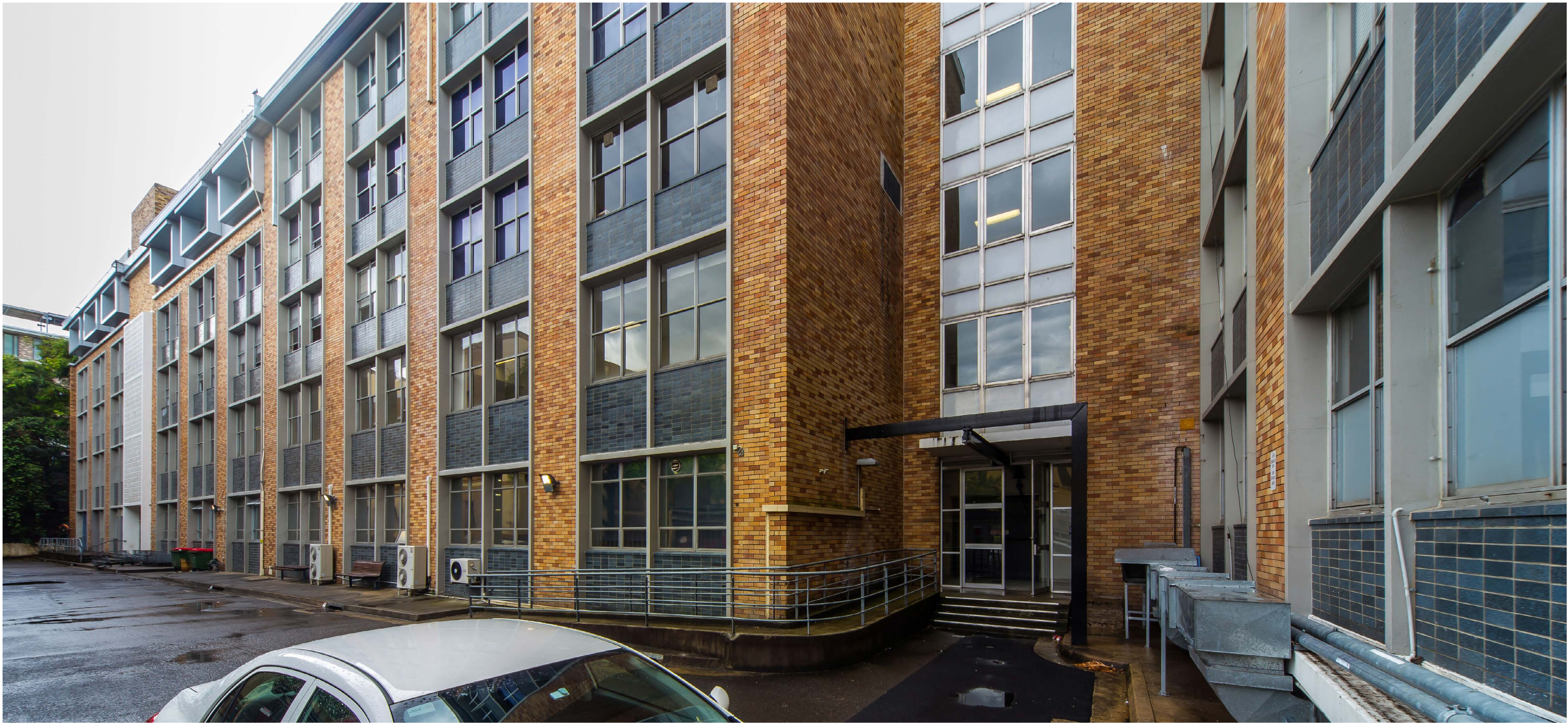
View of existing conditions taken from Rex Vowels courtyard looking towards the entry of Western Facade of the North Block.
