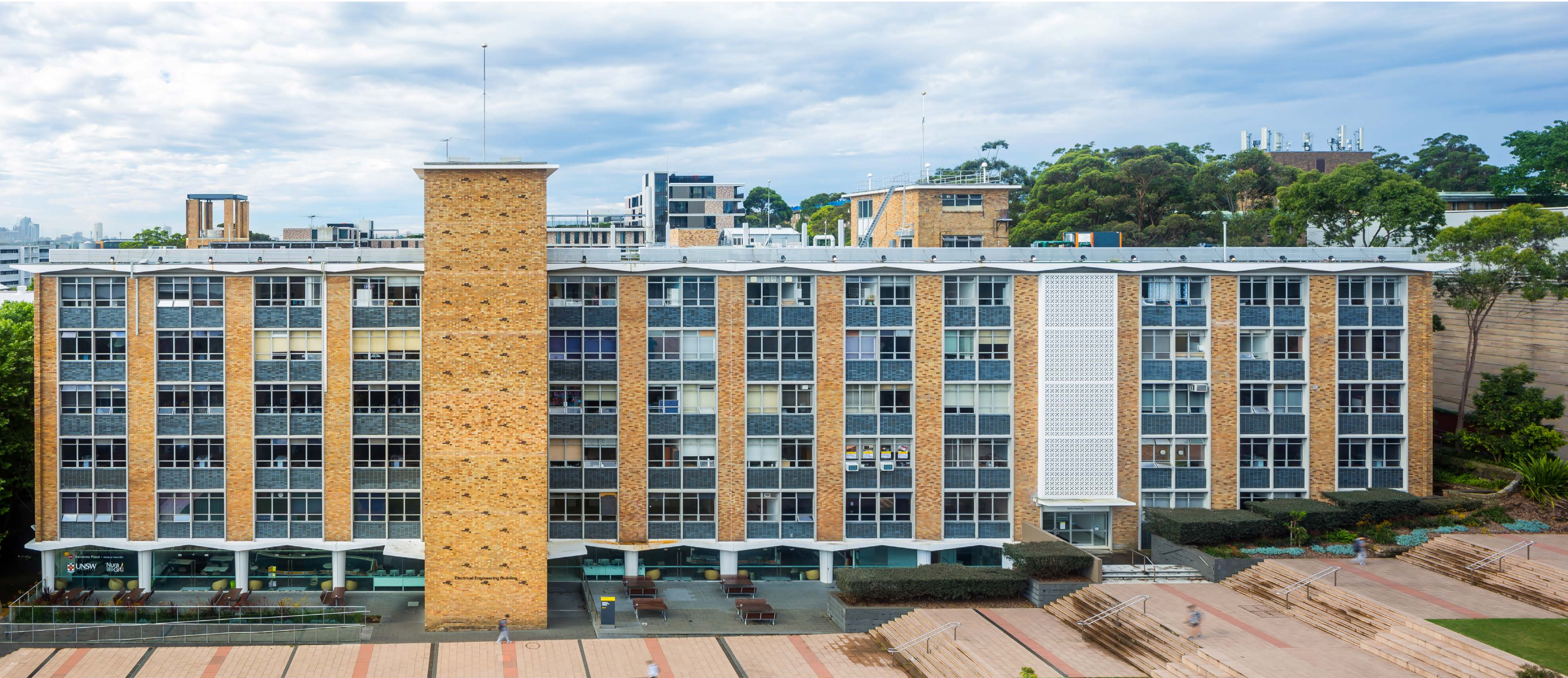
View of existing conditions taken from the roof of Mechanical Engineering Building looking towards the South Facade of the South Block.
