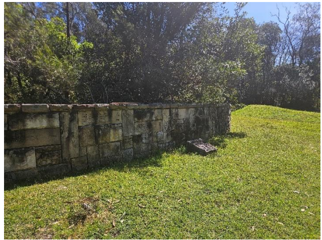
Figure 41 Sandstone wall located at the Oxford Falls Public School.
