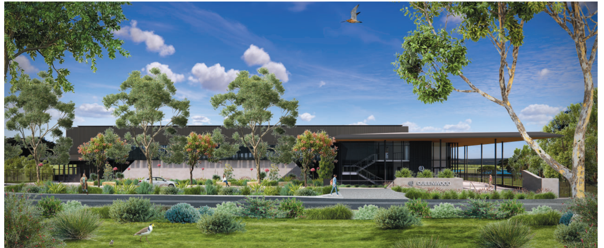
View of the front elevation of the Indoor Sport Hall facing Oxford Falls Road showing the use of lowered verandahs, sunshades, and varied materials to break up the extent of facade and lower the perceived bulk and scale of the building.
