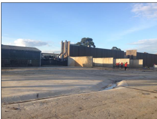
Figure 5-1 Stockpile yard and bays
