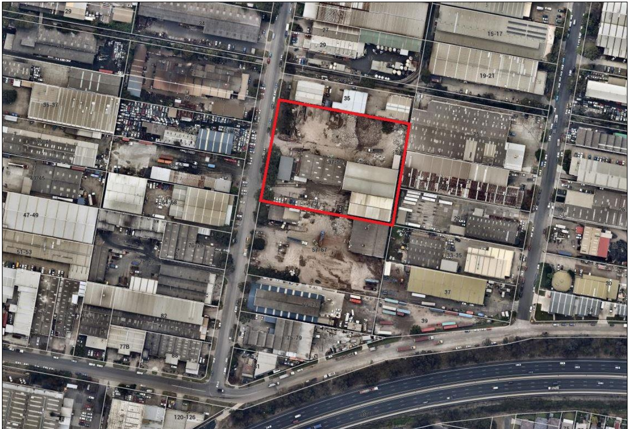
Figure 2-1 Existing Recycling Facility
