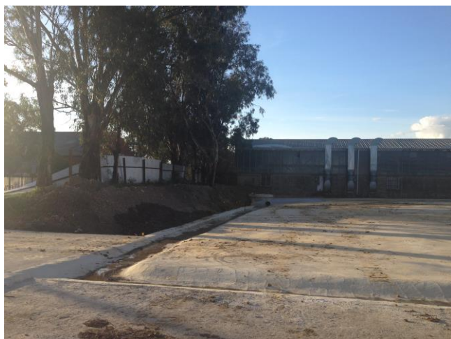
Figure 5-13 Drainage line in northern portion of site leading to sediment tank
