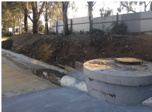
Figure 5-12 Sediment tank located in north-west corner of the site
