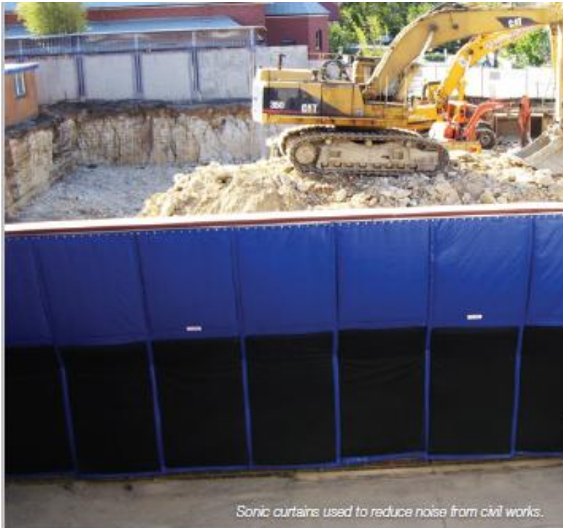
Figure 23: Example of Proposed Temporary Noise Barriers (2)
