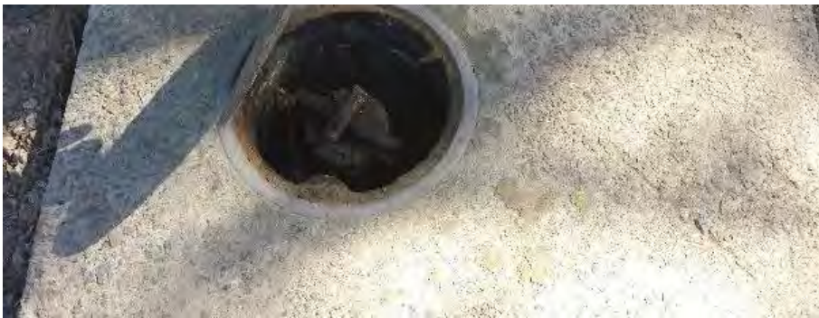
Photograph 13: Decommissioned UST fill points adjacent to southern driveway and office building.
