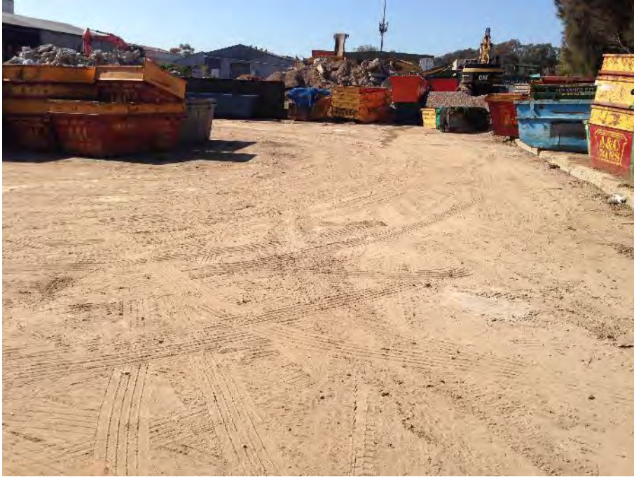
Photograph 5: Materials / storage bins on the Site
