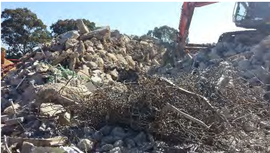
Photograph 6: Concrete rubble and metal stockpiles on the Site
