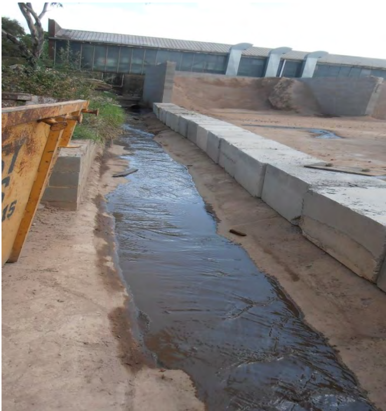
Photograph 12: Drainage line towards Gross Pollutant Trap (GPT) in north-western corner of the Site. GPT drains the northern portion of the Site.
