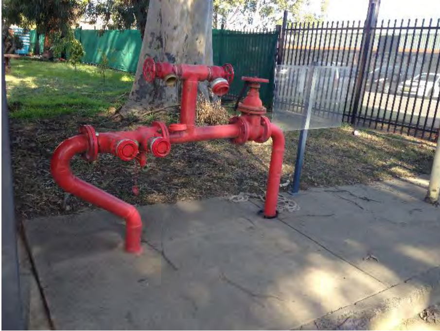
Photograph 11: Fire hydrant adjacent to southern driveway.
