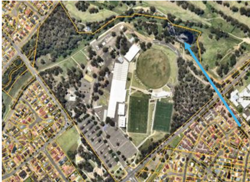
Figure 10 - Existing stormwater discharge location (Nearmap, 2024).
