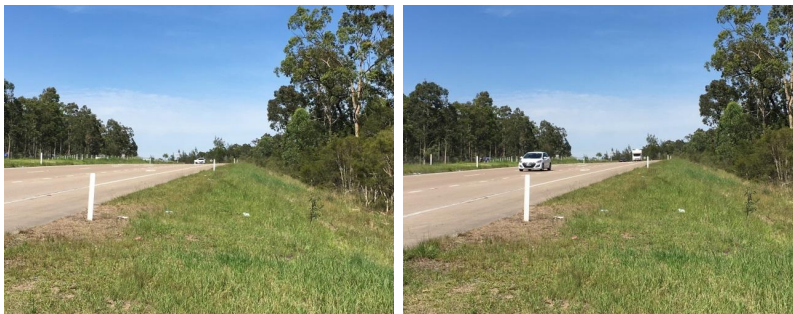
Figure 4-3 Sight distance observations across northbound vertical curve
