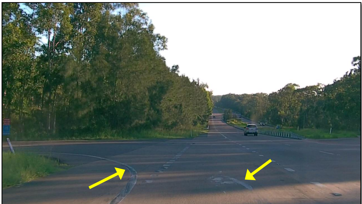
Photo 6: There are faded pavement markings (pavement turn arrows and edgeline) at the Italia Road intersection for the highway northbound left-turn lane.
