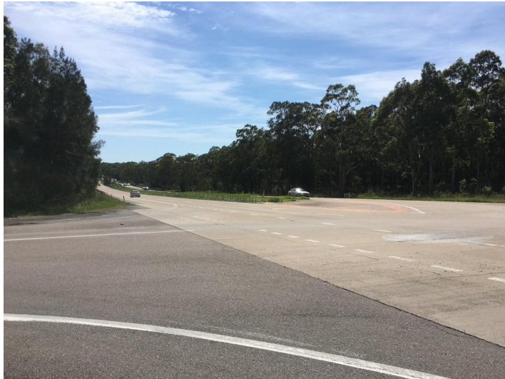
Figure 2-4 Italia Road intersection looking north to Karuah
