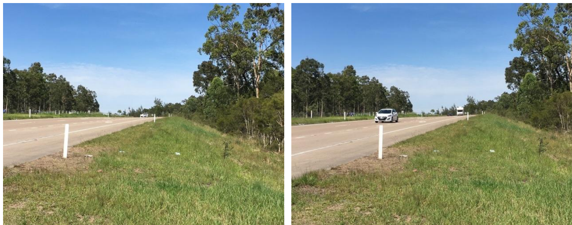
Figure 4-3 Sight distance observations across northbound vertical curve
