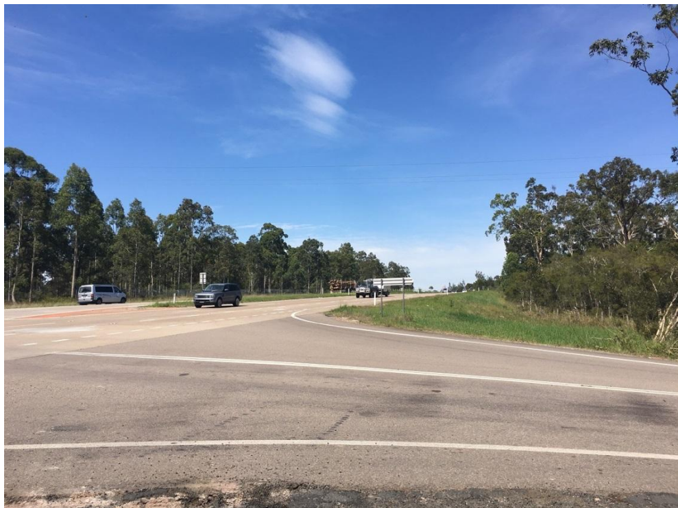
Figure 2-1 Pacific Highway approach to Italia Road
