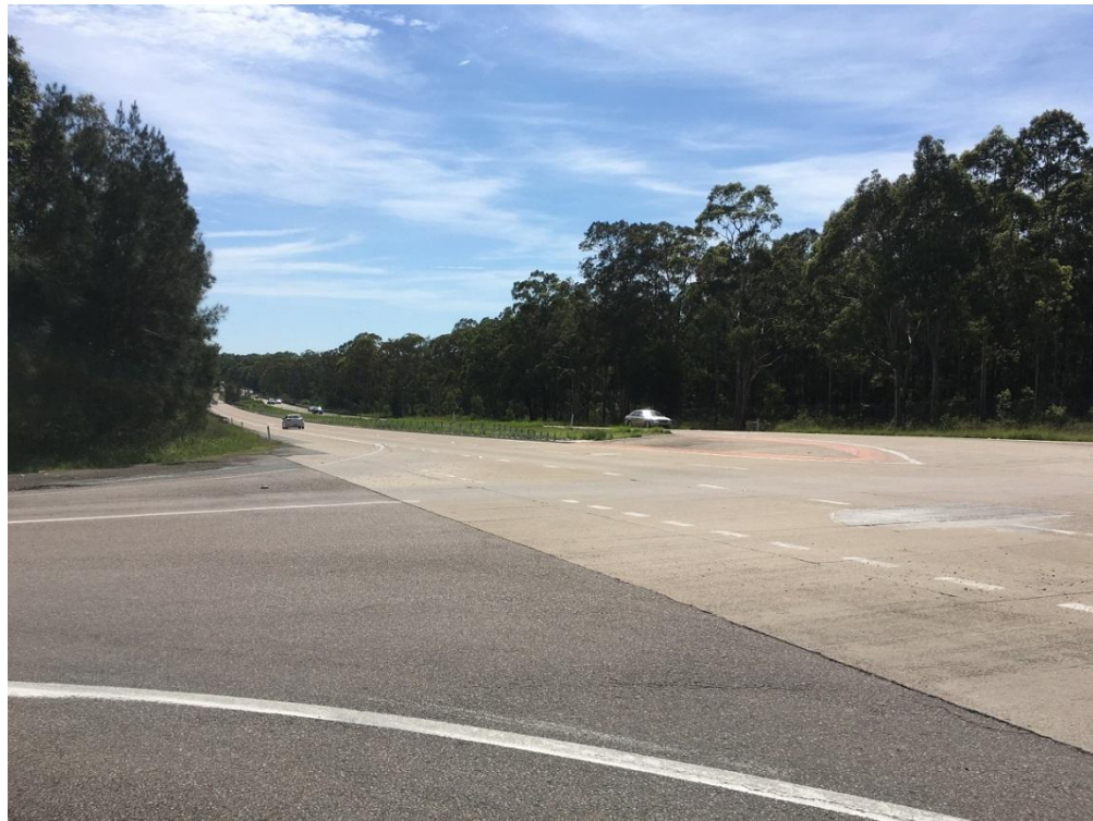
Figure 2-4 Italia Road intersection looking north to Karuah
