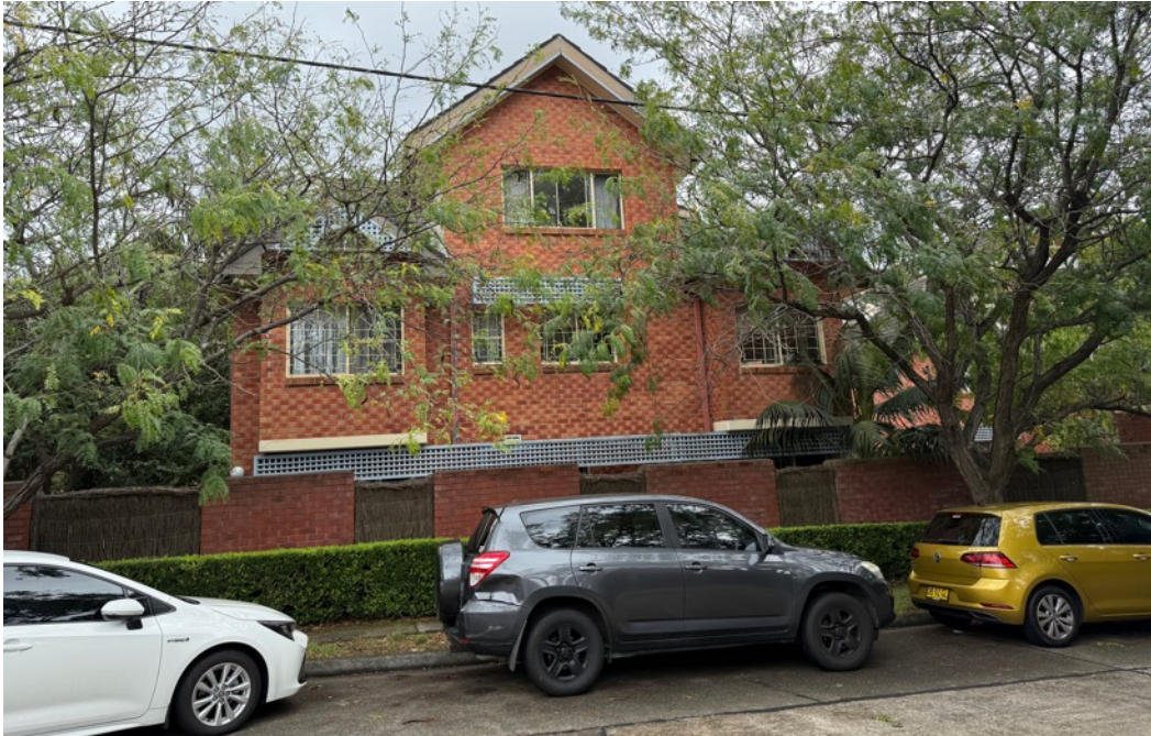
Figure 4: View of the site from Bertram Street.
