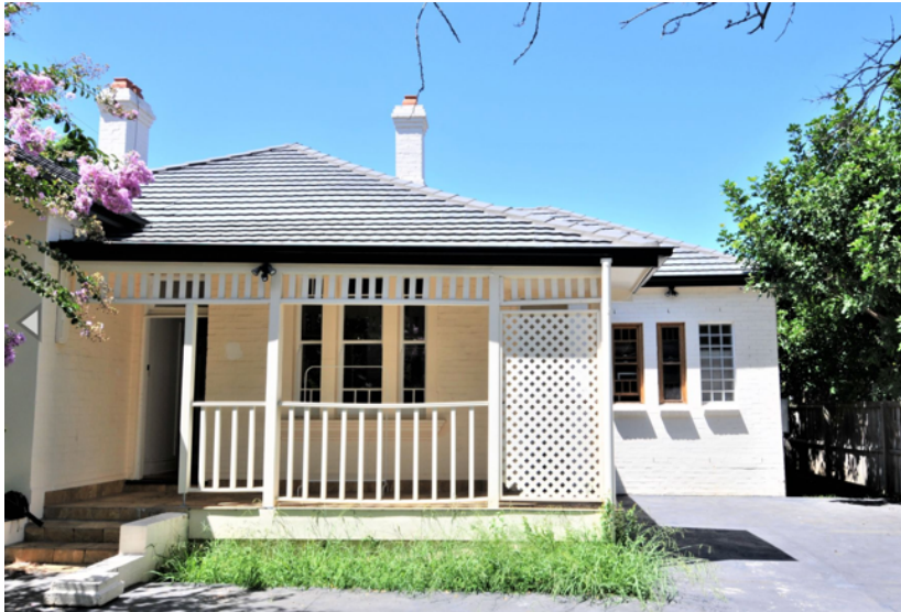
Figure 21: view of the item from Albert Avenue.
