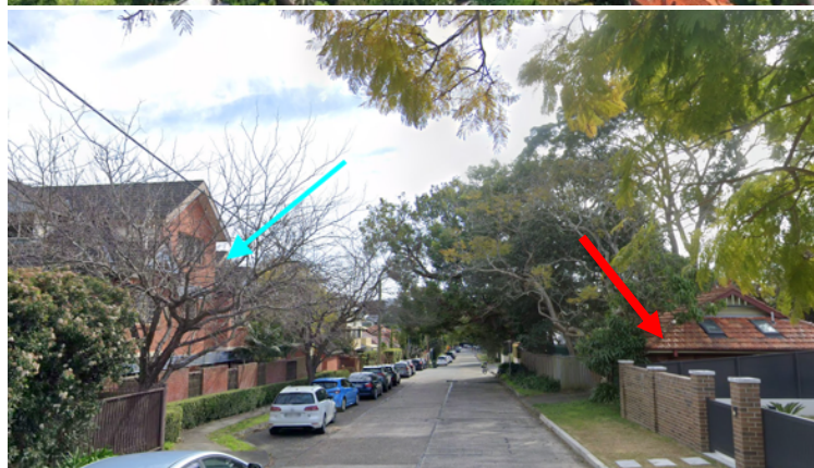
Figure 13: View along Bertram Street showing the site (blue arrow) and item red arrow.
