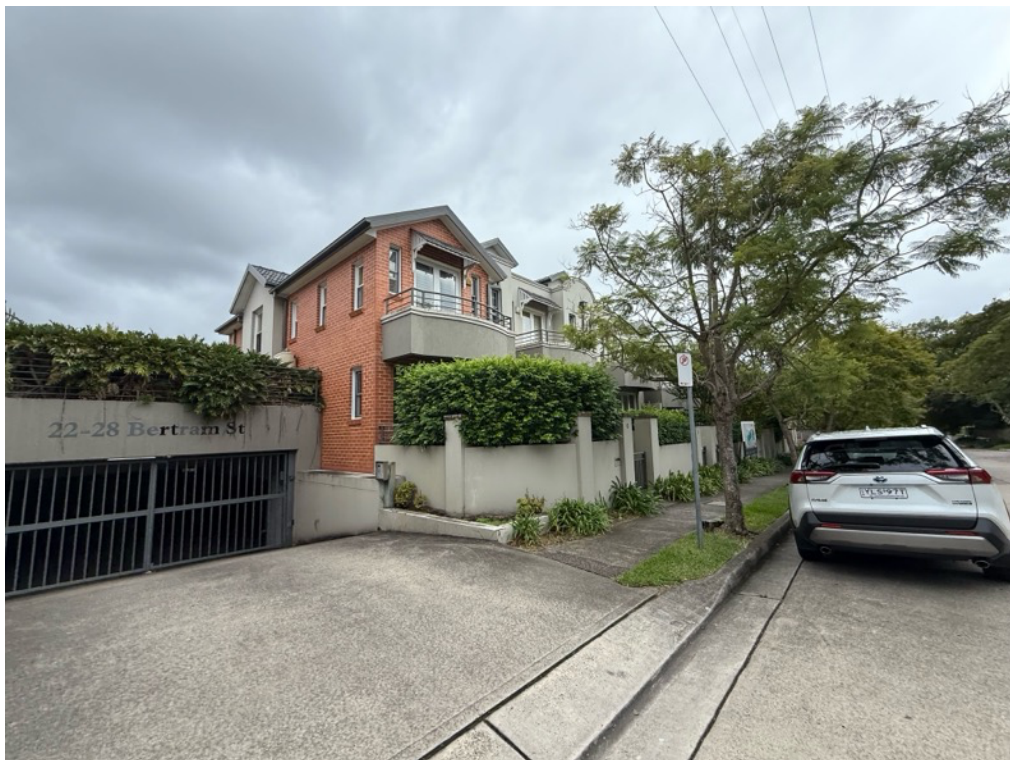
Figure 7: Modern duplex developments on the western side of Bertram Street.
