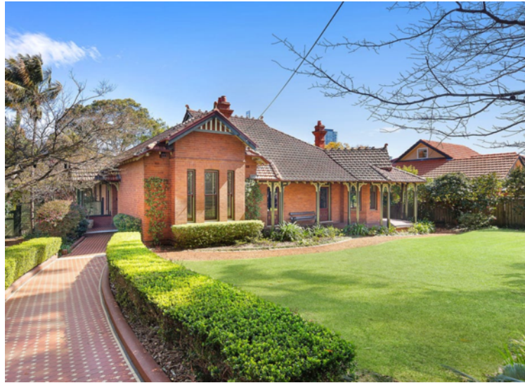
Figure 11: View of the item from Neridah Street.
