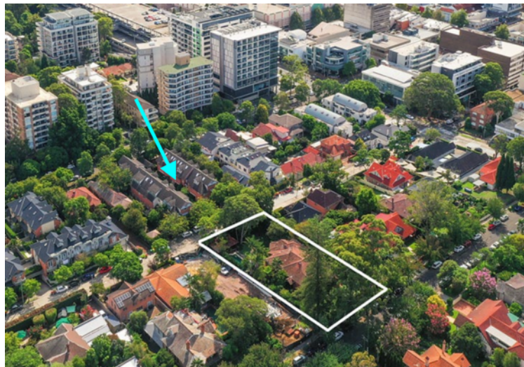
Figure 12: An oblique aerial photograph illustrating the relationship of the item to the site (blue arrow).
