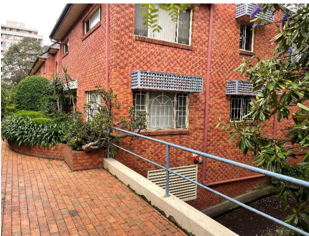
Figure 21 - View of the central courtyard over the basement access point, showing the depth of basement excavations.
