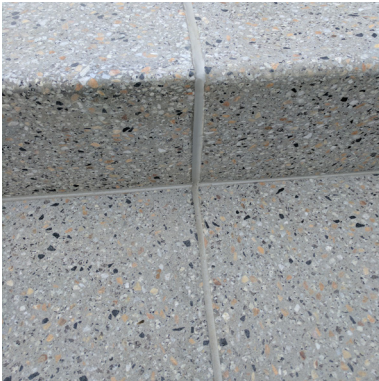
Auditoria Seating External Pavers Exposed Aggregate Finish
