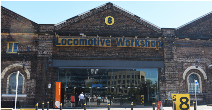
Existing photographs of Locomotive Workshop along Locomotive Street
