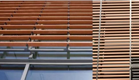
4. aluminium battens finished to match adjacent cladding
