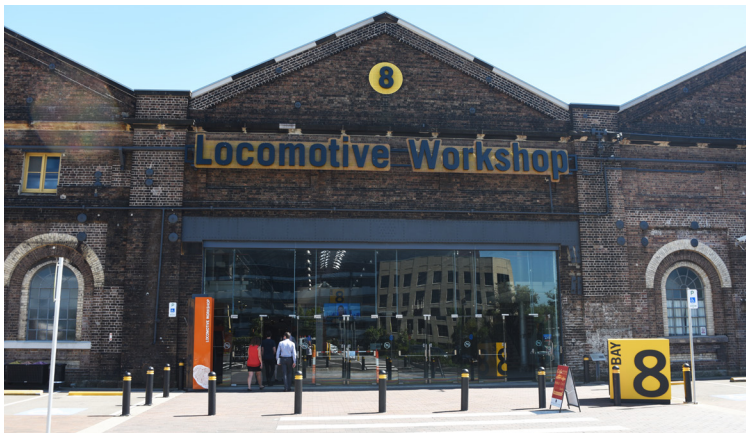
Locomotive Workshop - glazed entry on Locomotive Street
