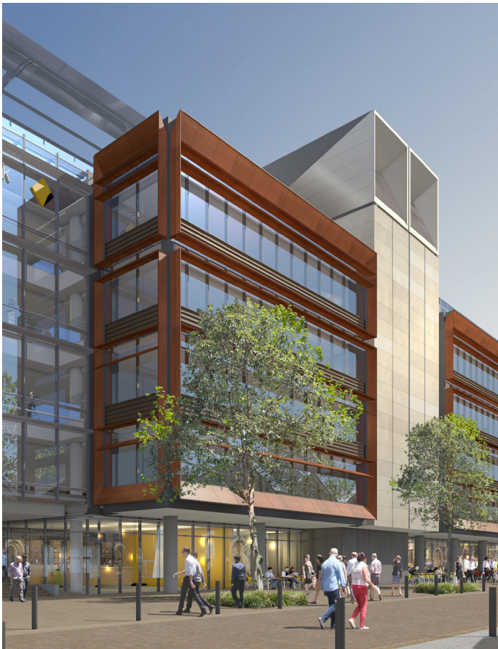
Image of B2 north facade showing horizontal articulation
