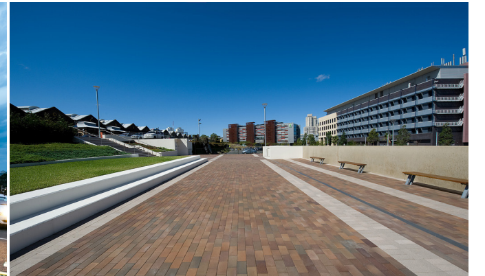
3. Biomedical building (1 Central Avenue) - to right
